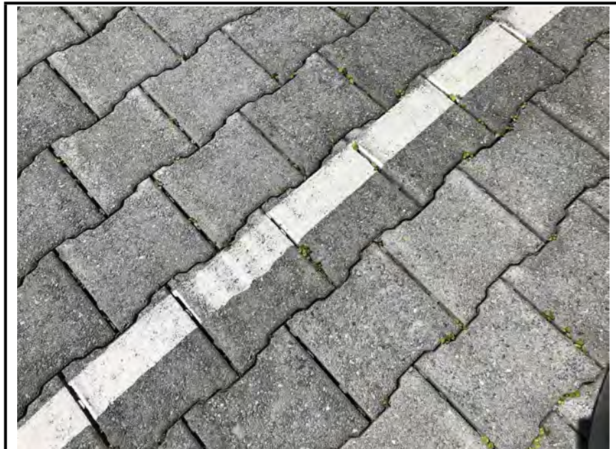
Photo #2: Close up view of the pavers.
