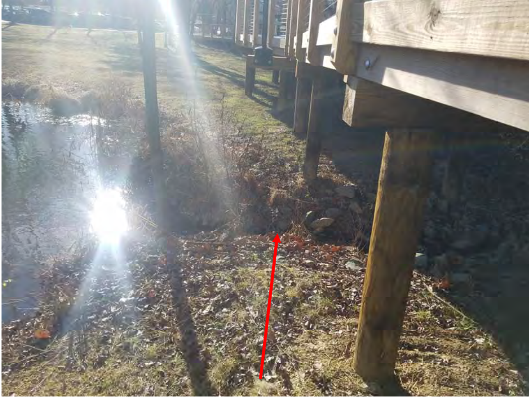
Control structure, riprap weir
