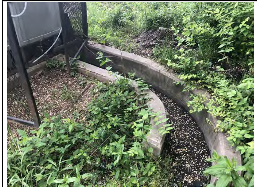
Photo #3: Inflow channel to the facility.
