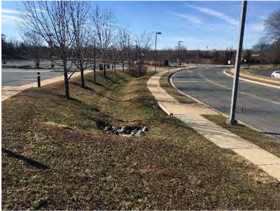
Inflow - COG Open Back, Grass Swale Conveyance
