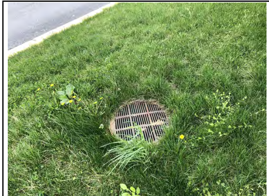
Photo #3: The grate outlet in the facility.
