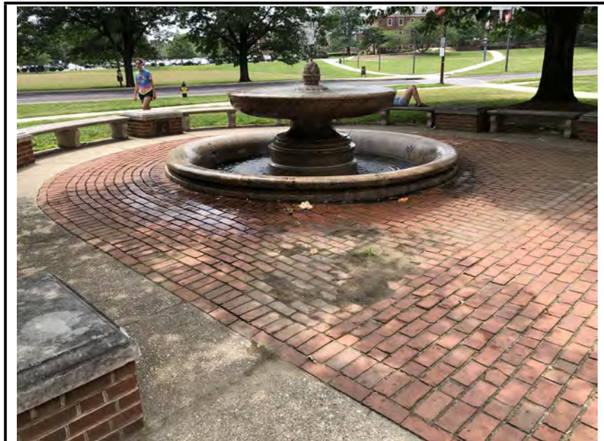
Photo #1: Missing brick pavers in pavement surface.
