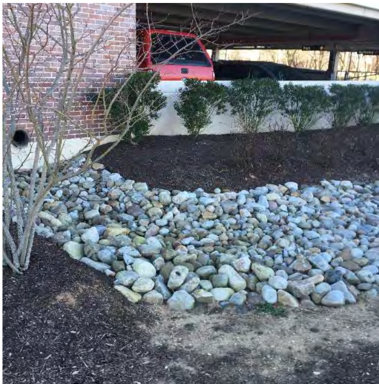
Inflow, Pipe from Parking Garage
