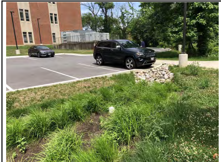
Photo #3: The riprap inflow that leads to the facility.
