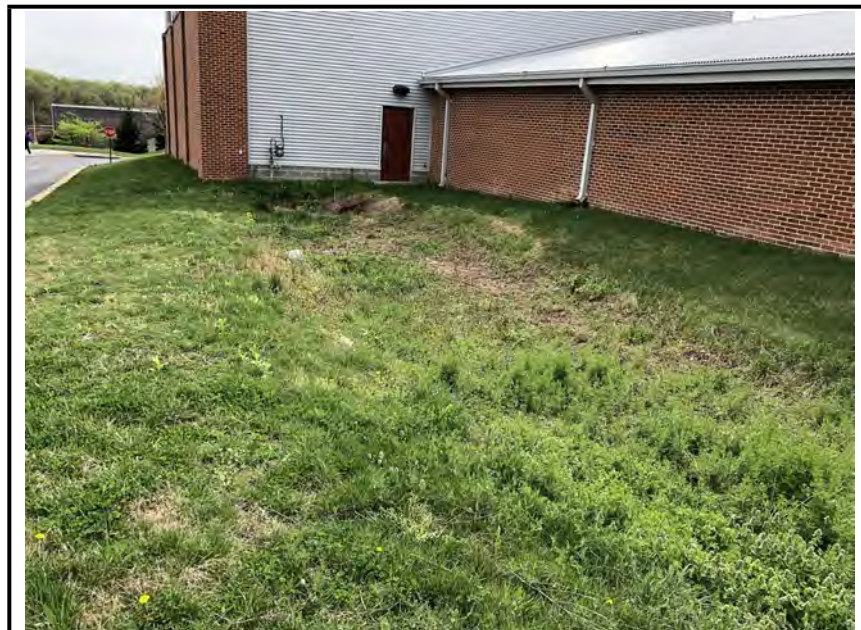
Photo #2: Vegetation inside the facility.
