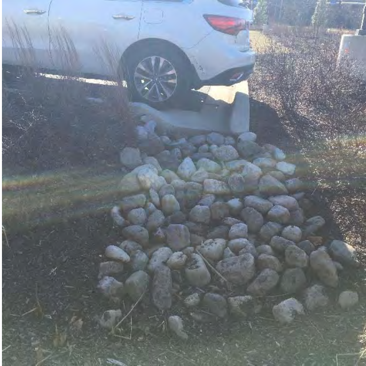
Inflow A - Curb cut from parking lot
