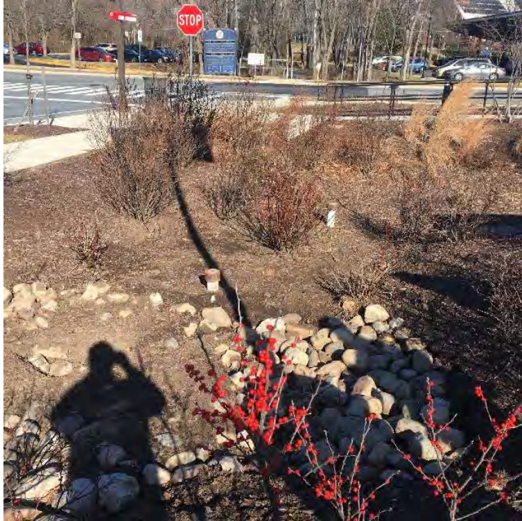
Overall B - Facing North, Cleanout
