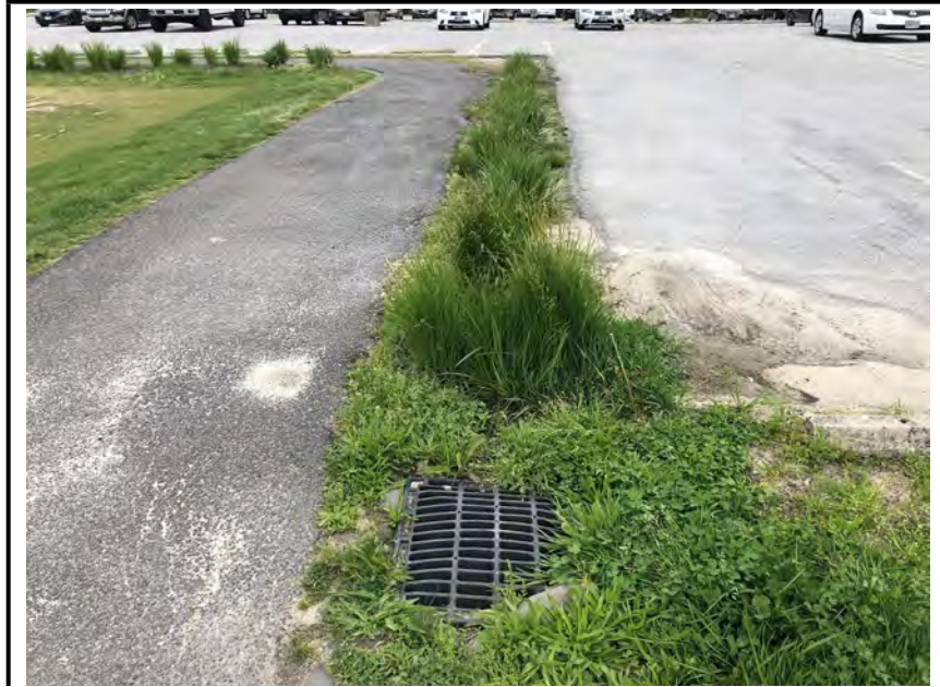
Photo #1: The pretreatment swale.
