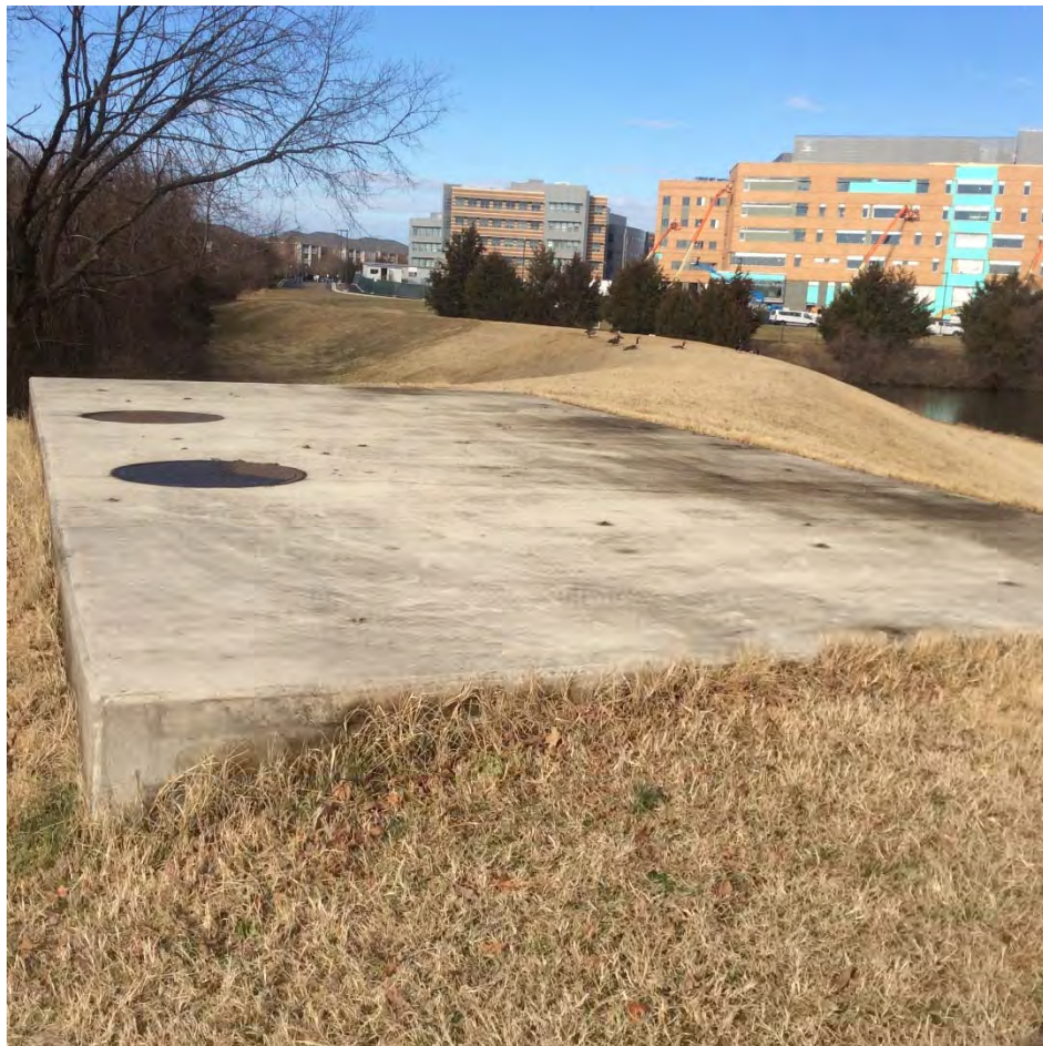
Control Structure Access
