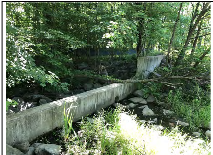
Photo #4: The outlet structure headwall.
