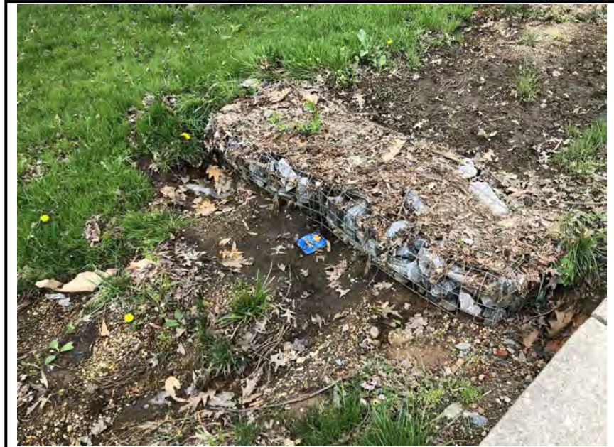
Photo #3: Gabion weir.
