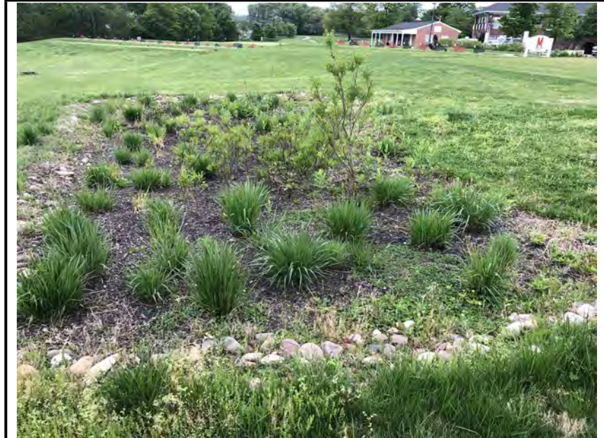
Photo #3: The vegetation within the facility.
