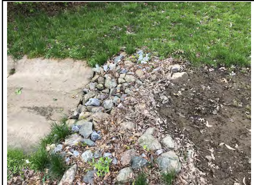
Photo #5: Rip rap to outflow.
