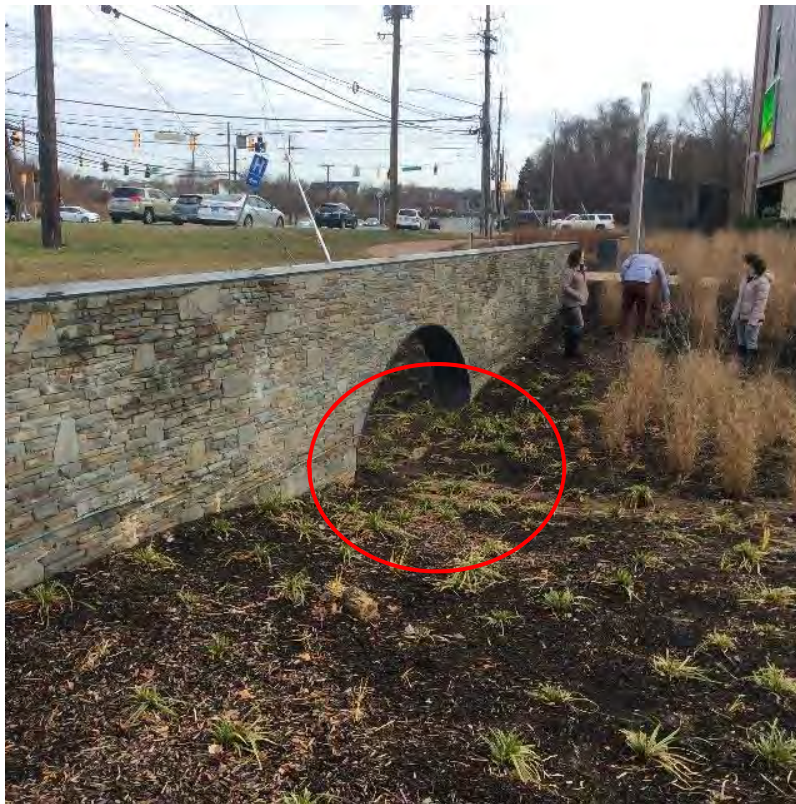
Arch located within BMP, BMP low point
