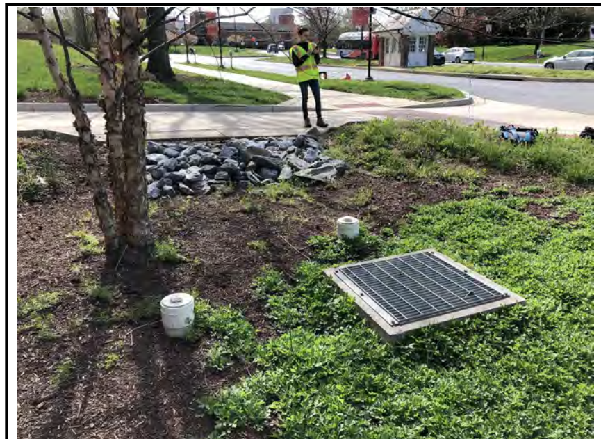
Photo #2: View of the facility.
