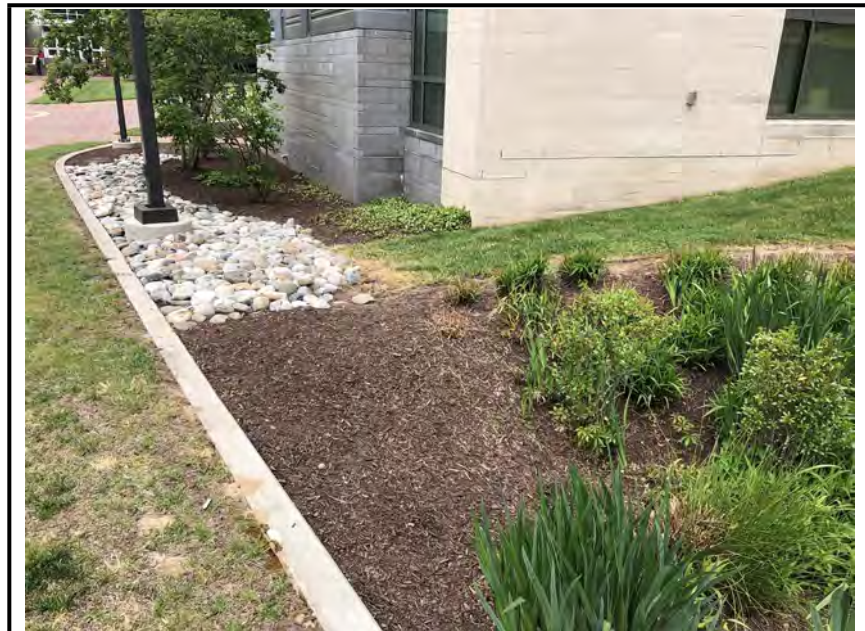
Photo #4: Curb lines the outside edge.
