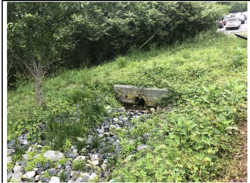
Photo #1: The inflow culvert to the facility.
