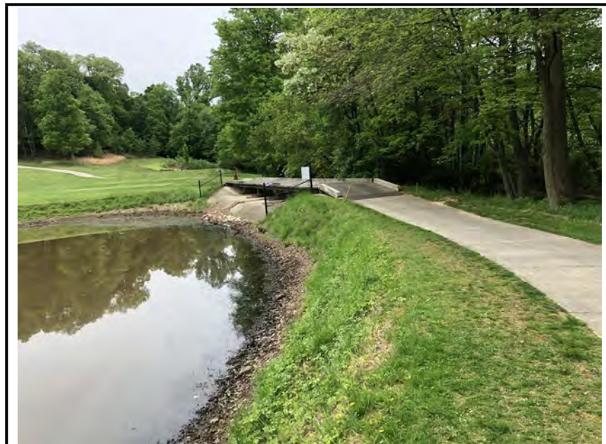
Photo #2: Front of the dam.
