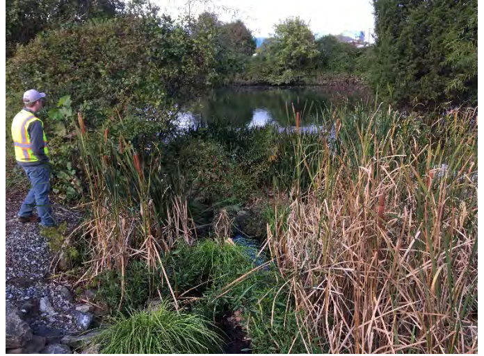
Figures 9-12 – Photos of the silted in inflow at the point where the two 30" pipes and one 15" pipe enter Gudelsky Pond.
