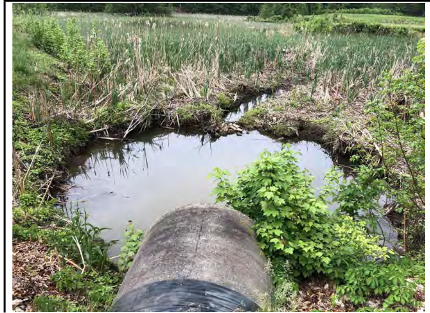
Photo #3: Small ponded area at inflow pipe.
