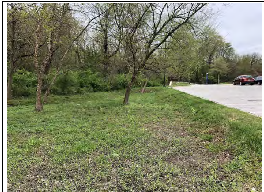
Photo #2: The filter area of the facility.
