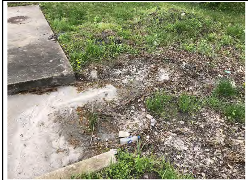
Photo #1: The curb cut through which runoff enters the facility.
