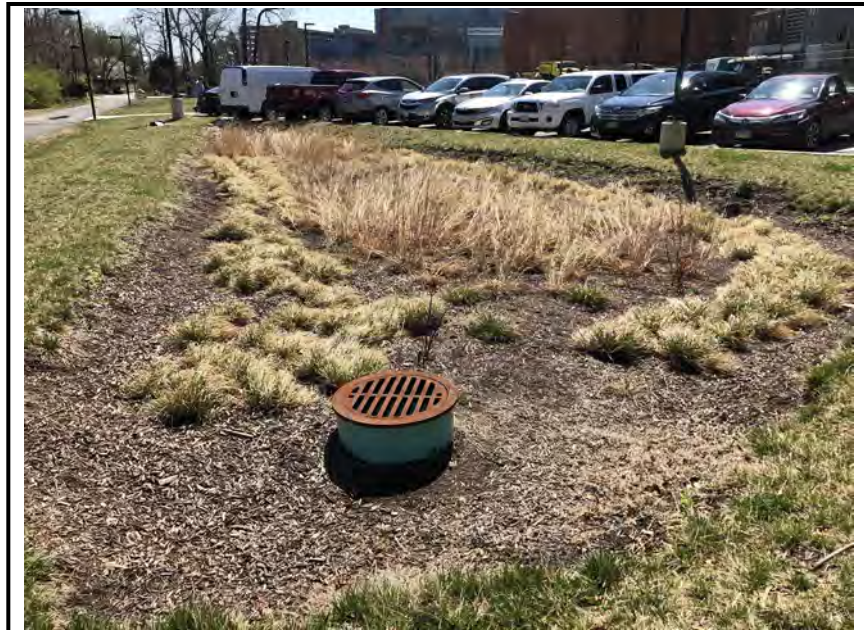
Photo #3: The riser outfall structure.
