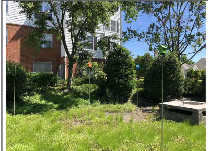
Photo #3: The outfall structure.
