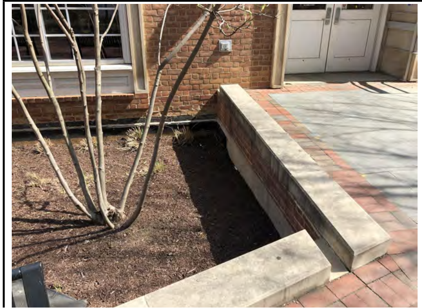
Photo #1: Curb cuts that lead into one of the forebays.
