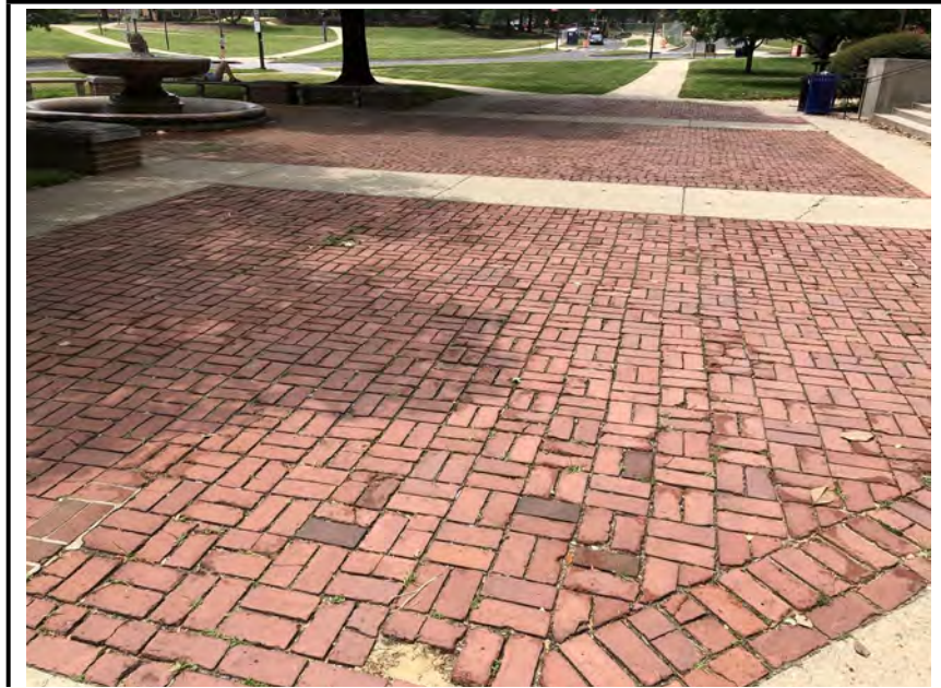
Photo #1: Missing brick pavers in pavement surface.
