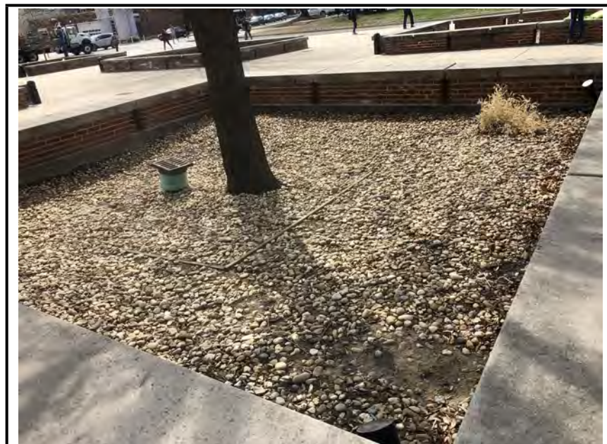
Photo #1: View into the facility.
