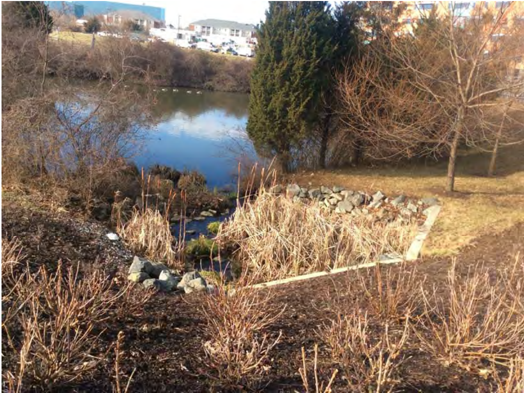
Forebay, Cattail Growth
