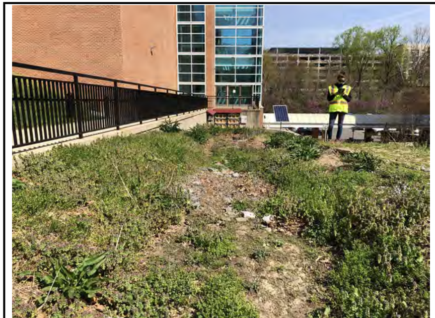
Photo #3: View into the facility.
