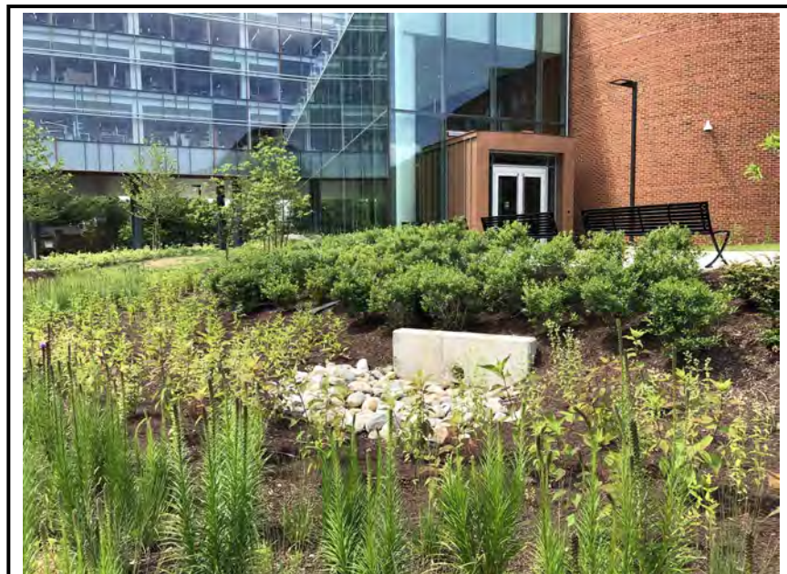
Photo #4: Inflow headwall that is lower than the filter bed area.
