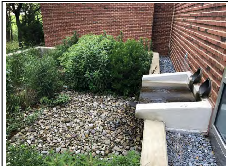
Photo #1: The riser outlet structure shared with CH-1
