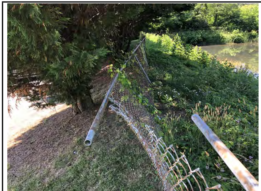
Photo #2: A section of broken fence.
