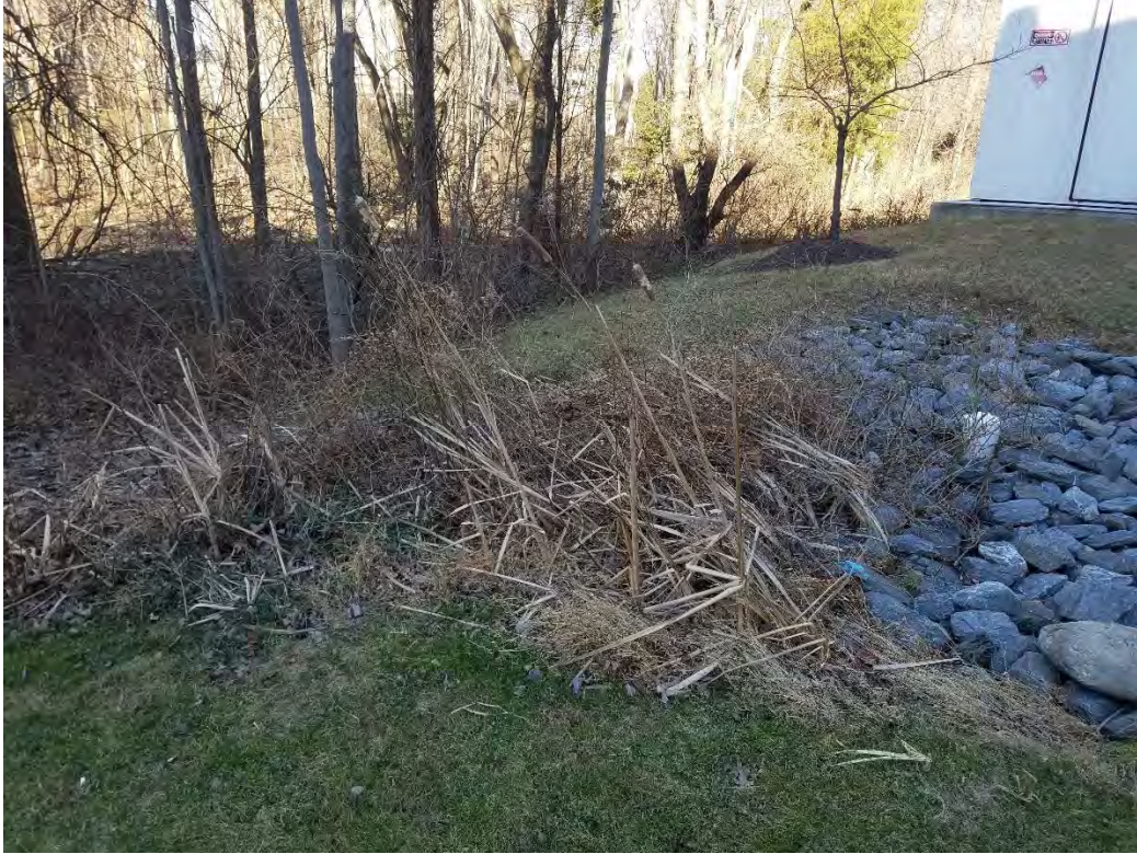
Overflow and overgrown vegetation
