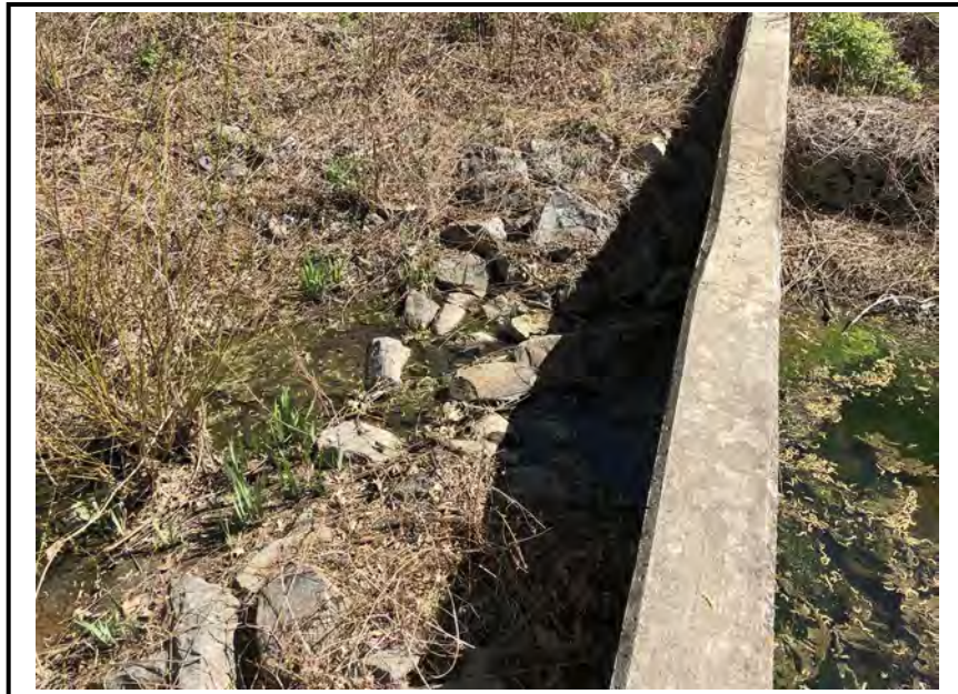
Photo #3: Outfall of flowsplitter, algae, debris present.
