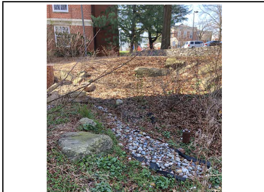
Photo #4: Stone inflow path into the facility.
