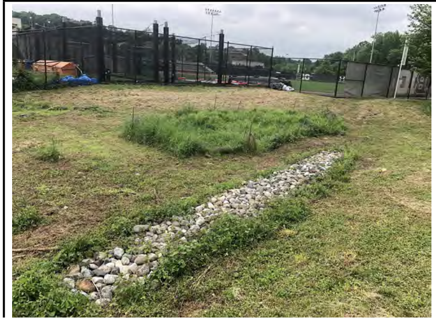
Photo #1: A strip of riprap that has no clear purpose.
