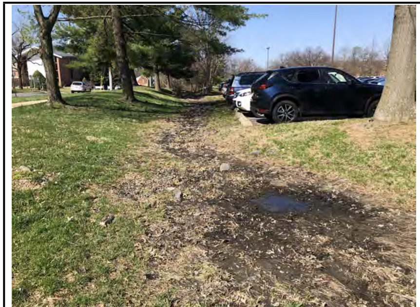
Photo #2: The pretreatment riprap channel.
