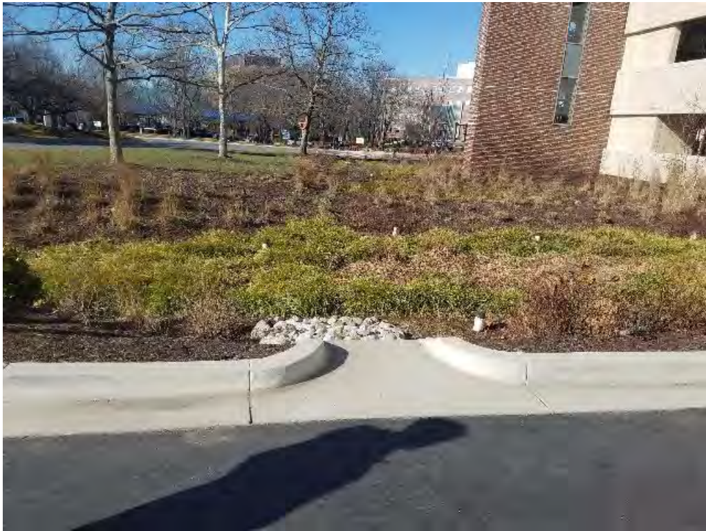
Inflow A, Curb Cut
