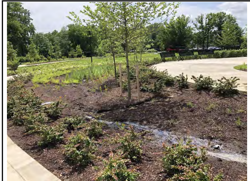
Photo #1: Erosion and standing water inside the inflow swale.
