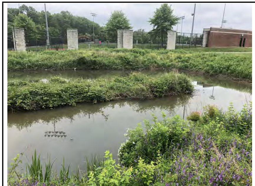
Photo #2: Possible forebay area. No weir is visible.
