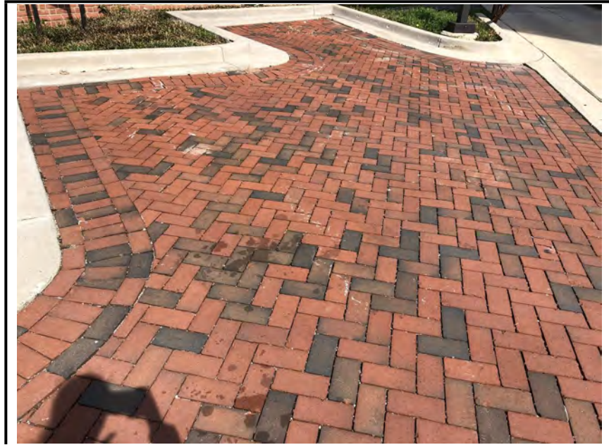
Photo #3: Stains on the pavers.
