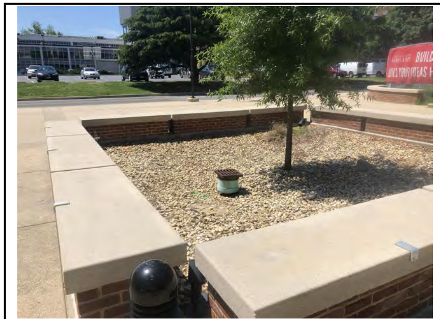
Photo #1: Close view of the filter bed.
