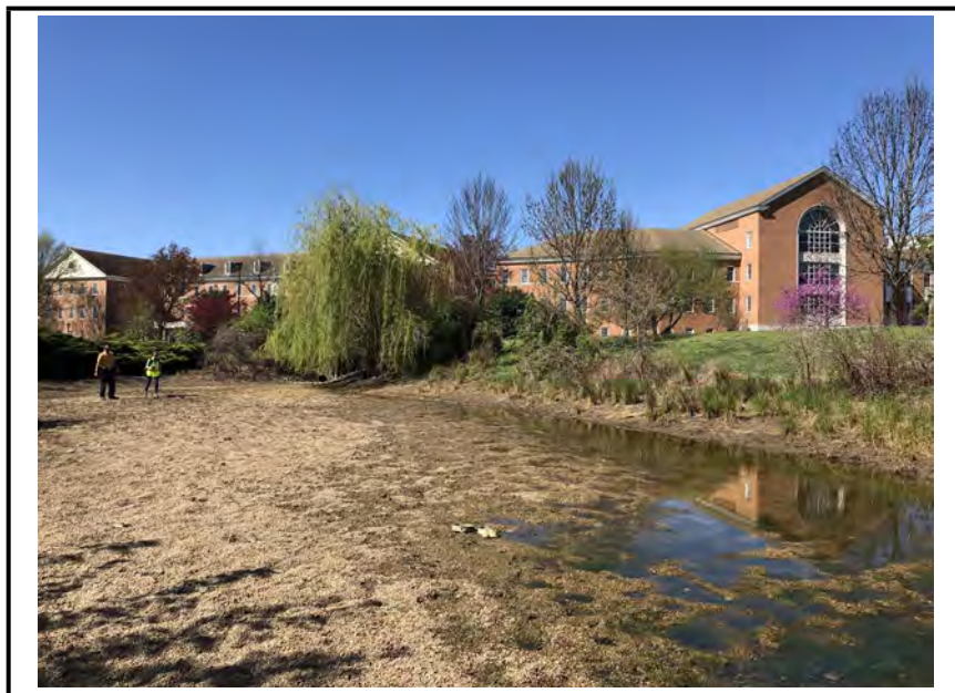
Photo #10: Sand filter area, ponding shown.
