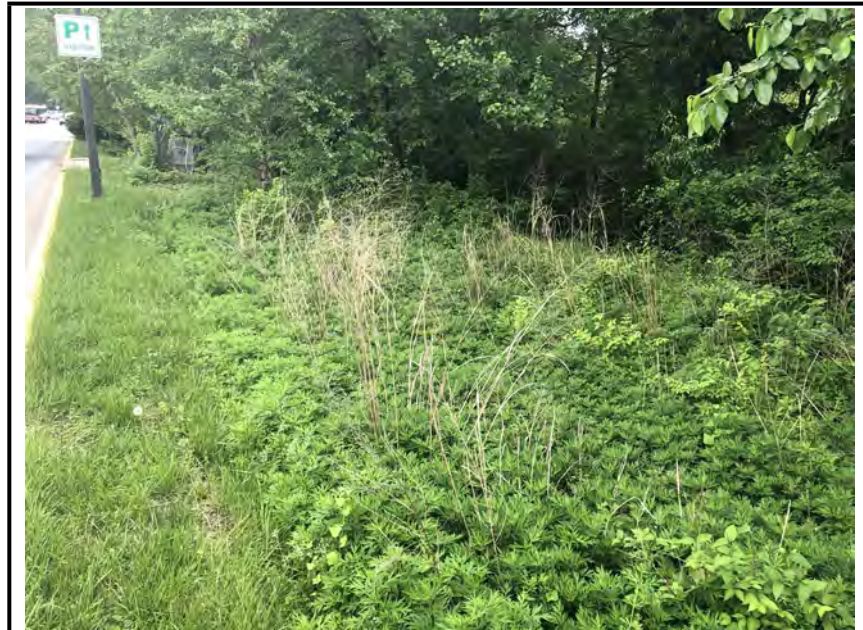
Photo #1: View of the overgrown filter area.
