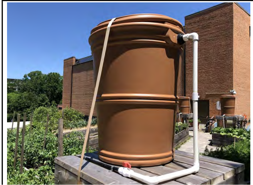
Photo #1: One of the 50-gallon rain barrels that store water for irrigation.
