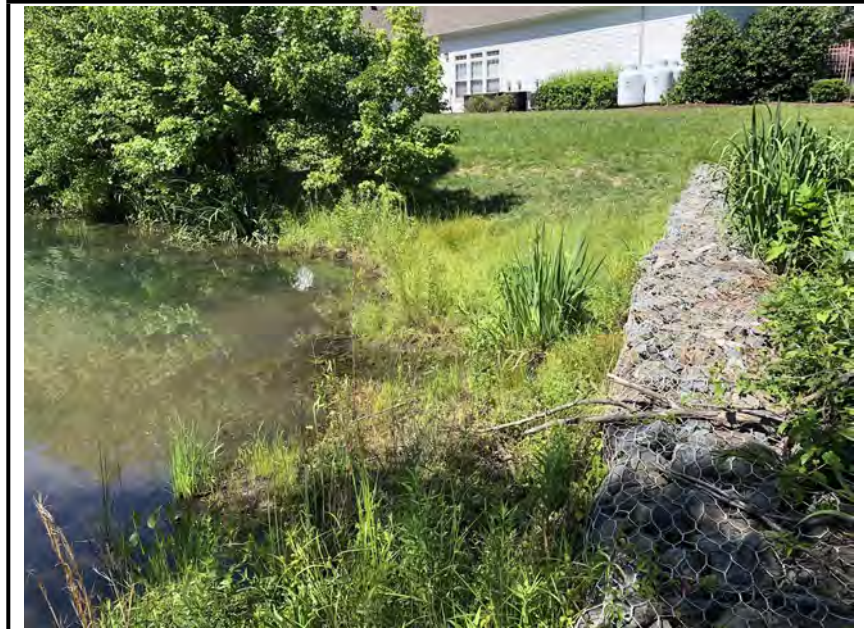
Photo #3: The gabion weir that separates the forebay from the facility.
