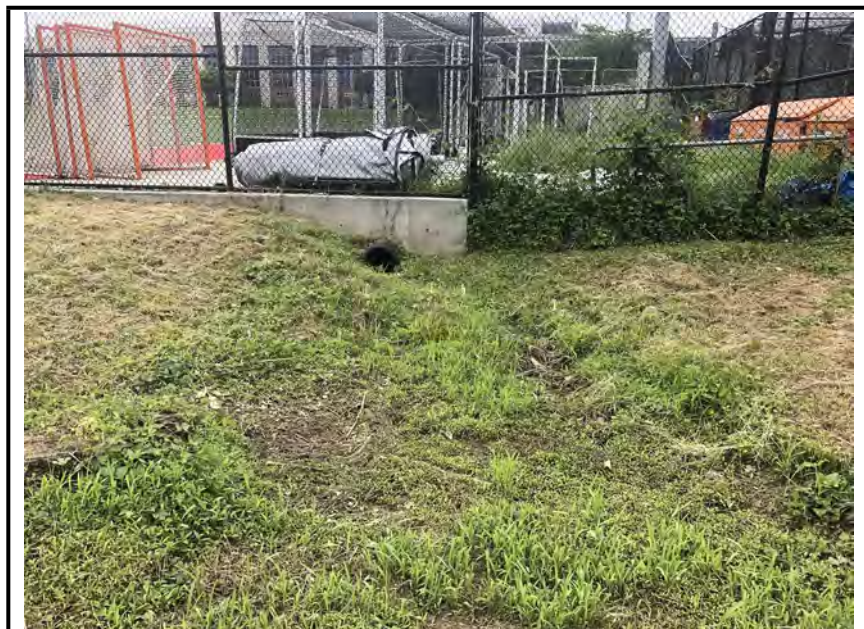
Photo #4: Inflow pipe and channel.
