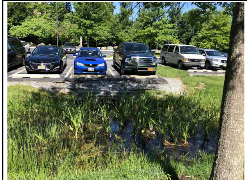
Photo #1: Standing water in the swale.
