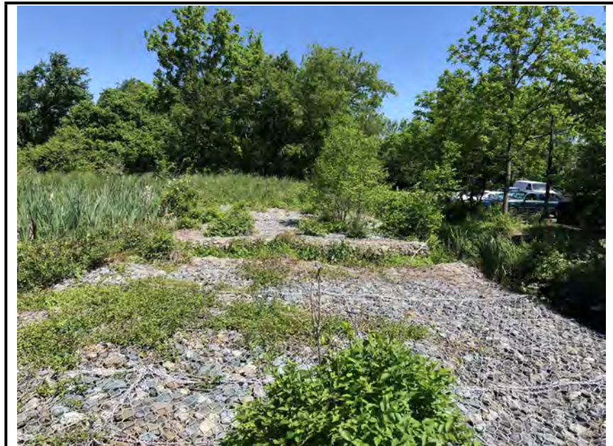
Photo #4: The gabion weir that flows into the swale.
