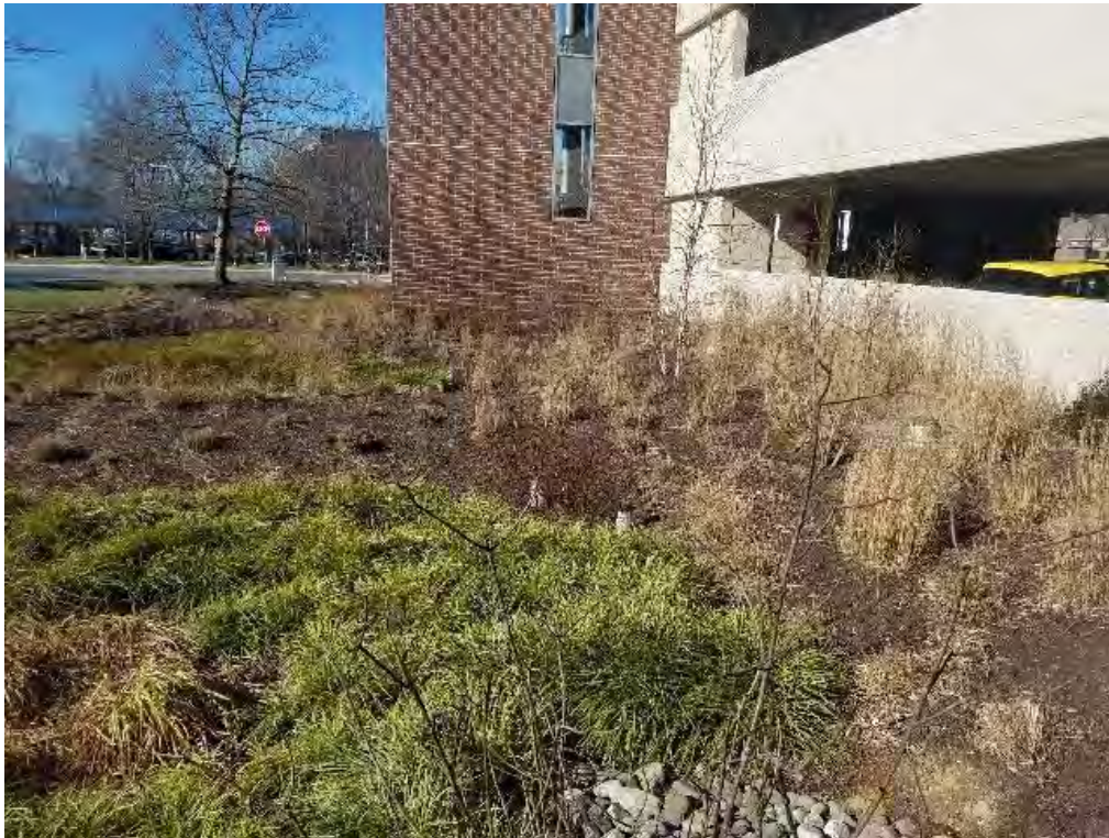
Overall Facing North
