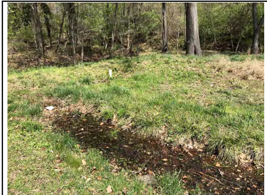
Photo #1: Standing water in the forebay.
