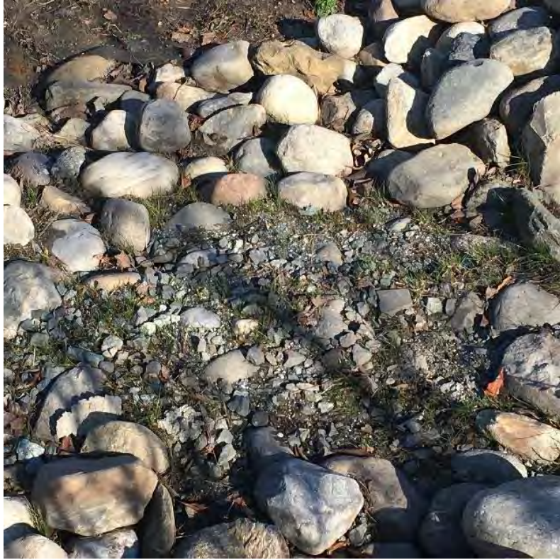
Gravel within Riprap
