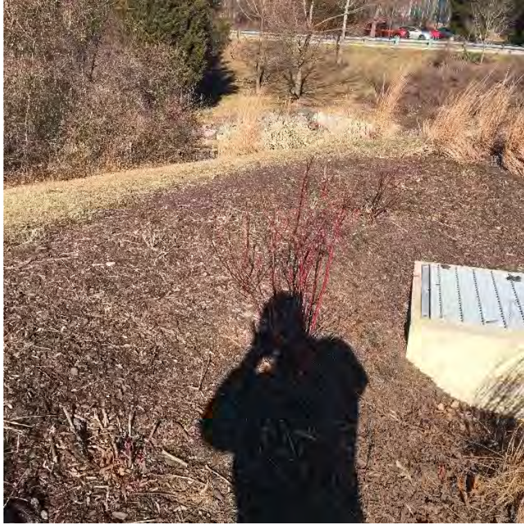
Embankment, Overflow Device
