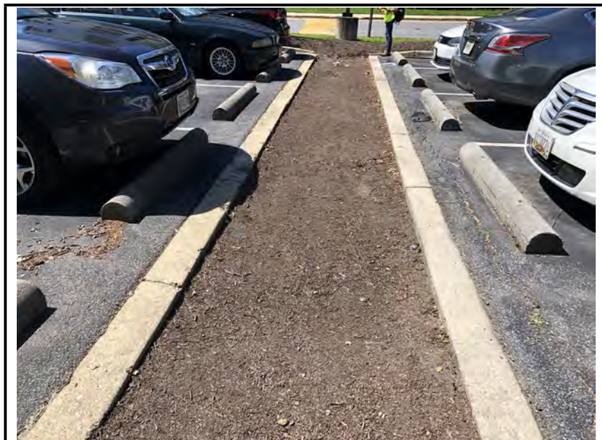
Photo #2: The unvegetated end of the facility.
