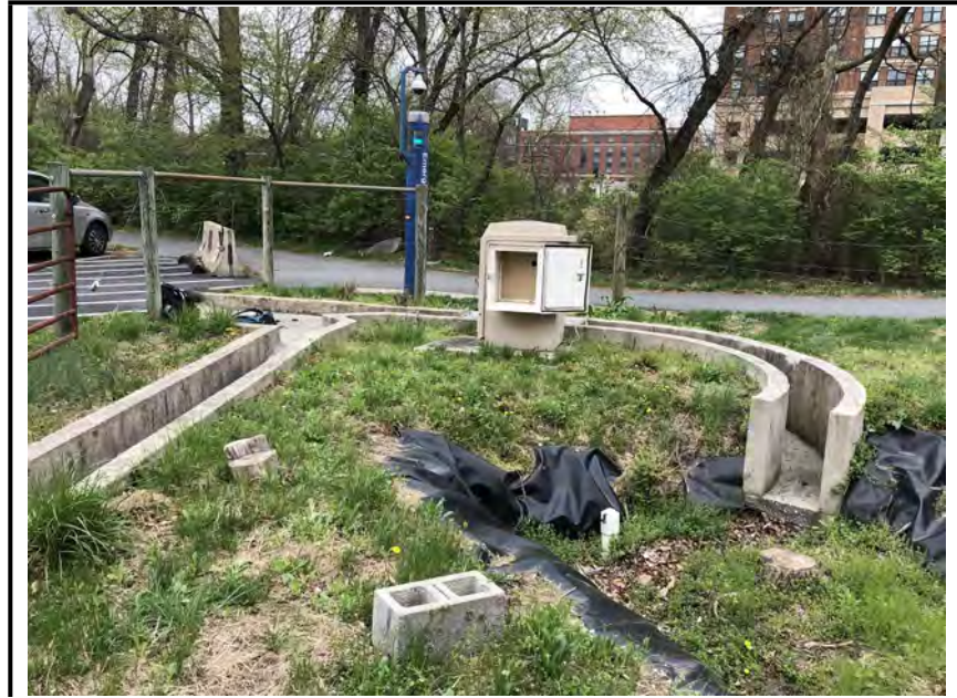
Photo #5: The inflow channels of both facilities.
