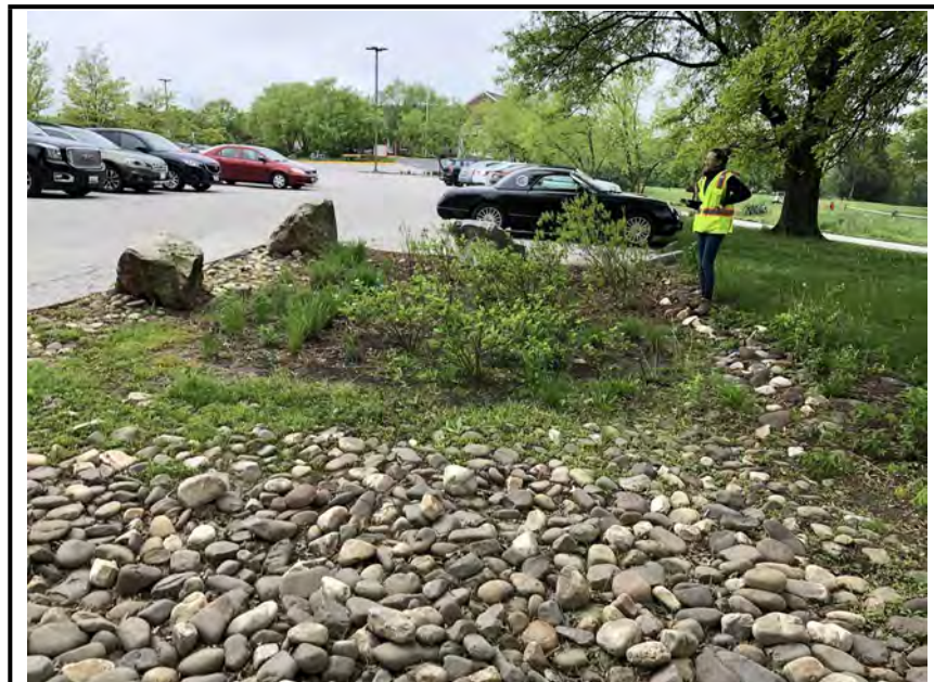
Photo #2: Pretreatment stage of the facility.
