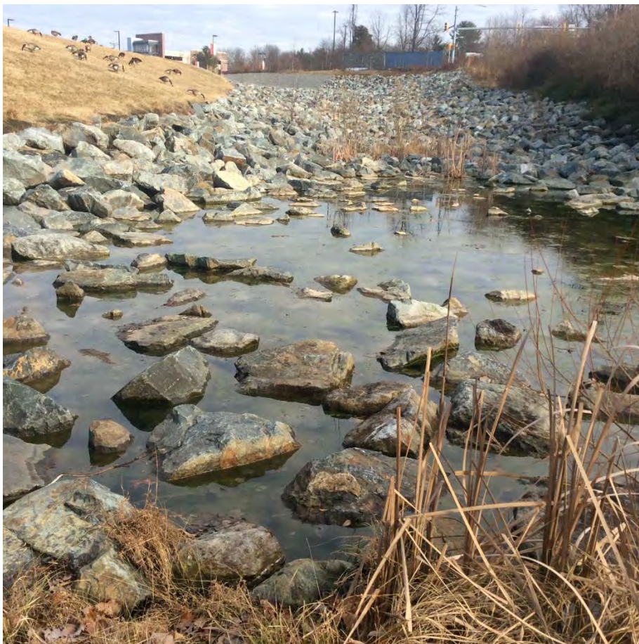
Emergency Spillway, standing water at end of spillway
