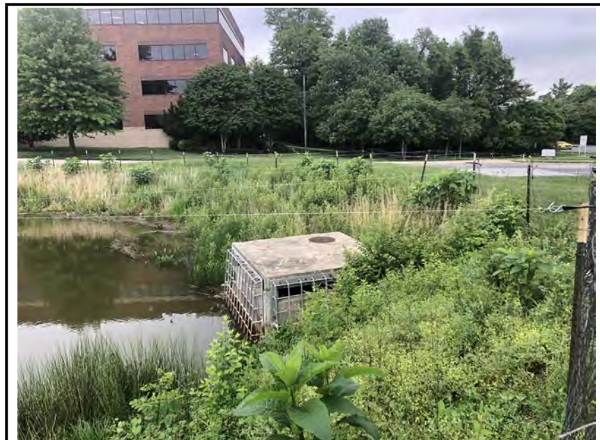
Photo #2: The outfall structure. Water is at the overflow level.
