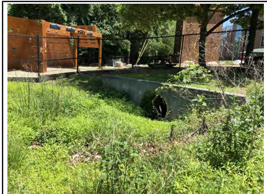
Photo #4: The outfall structure.
