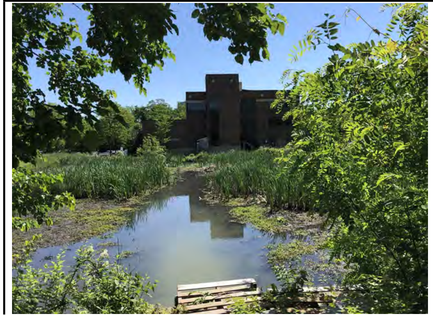
Photo #3: View into the facility from the inlet point.
