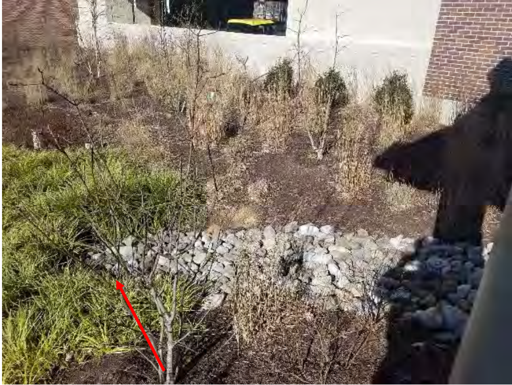
Inflow - Pipe from Parking Garage
