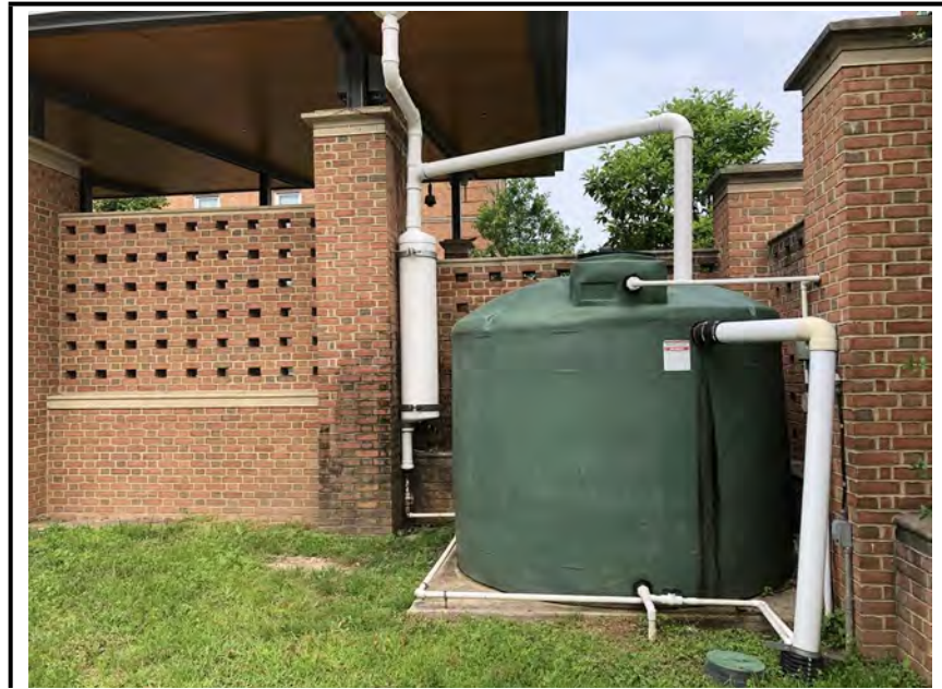
Photo #1: The rainwater harvesting facility.
