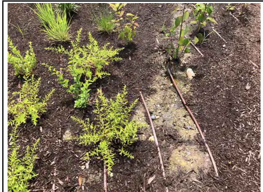
Photo #3: Exposed irrigation lines inside the facility.
