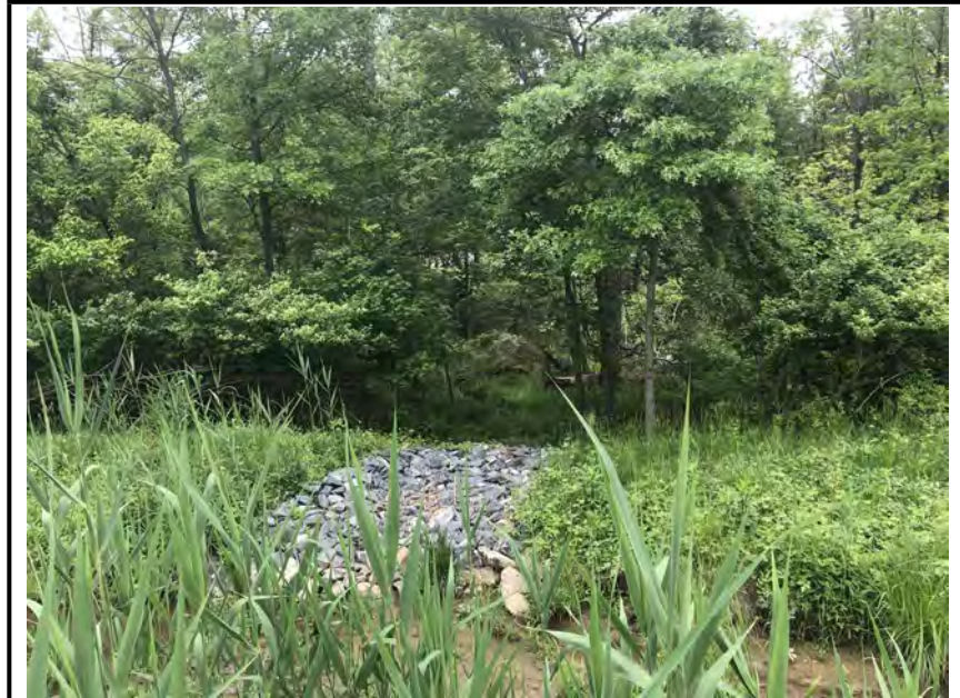
Photo #3: The riprap spillway.
