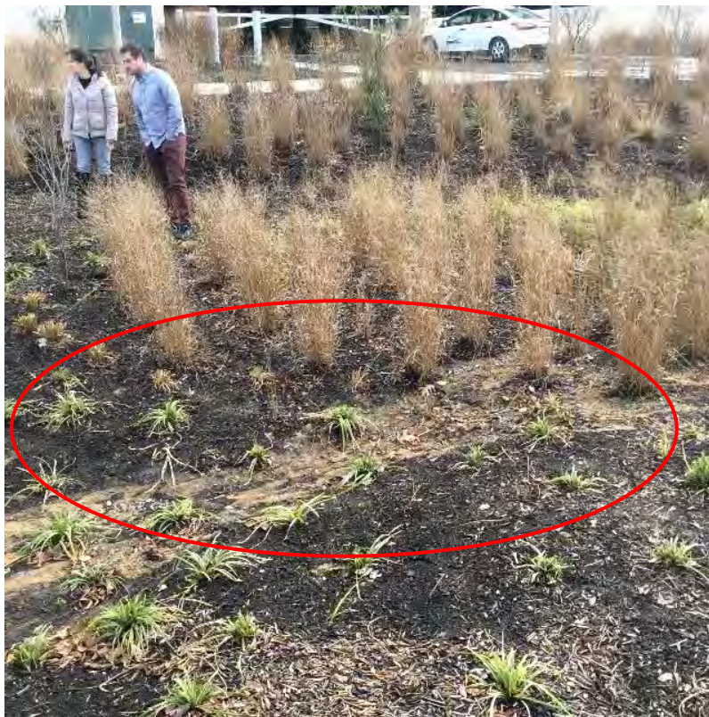
Erosive flow within BMP conveyance
