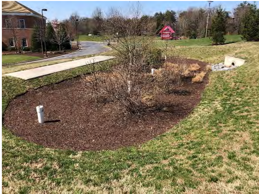
Photo #1: View from above the facility.
