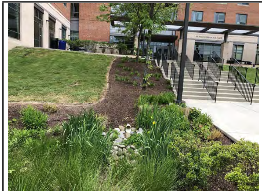
Photo #1: Outlet structure flush with the mulch elevation.
