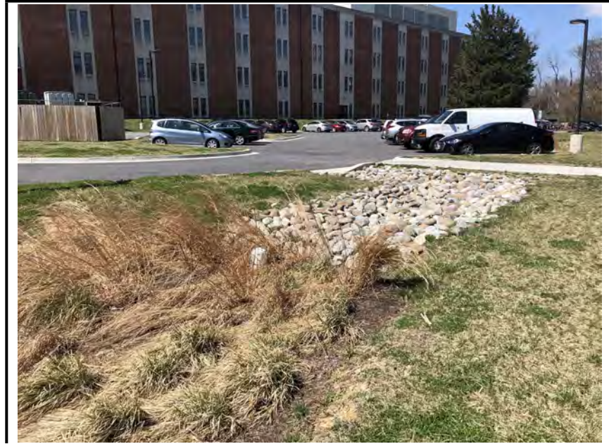
Photo #3: The riprap inflow channel.
