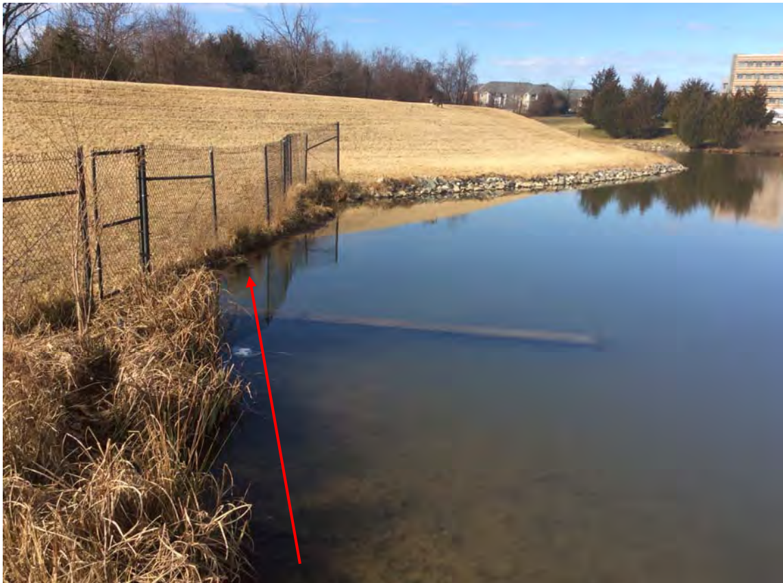
Low flow Device, Submerged
