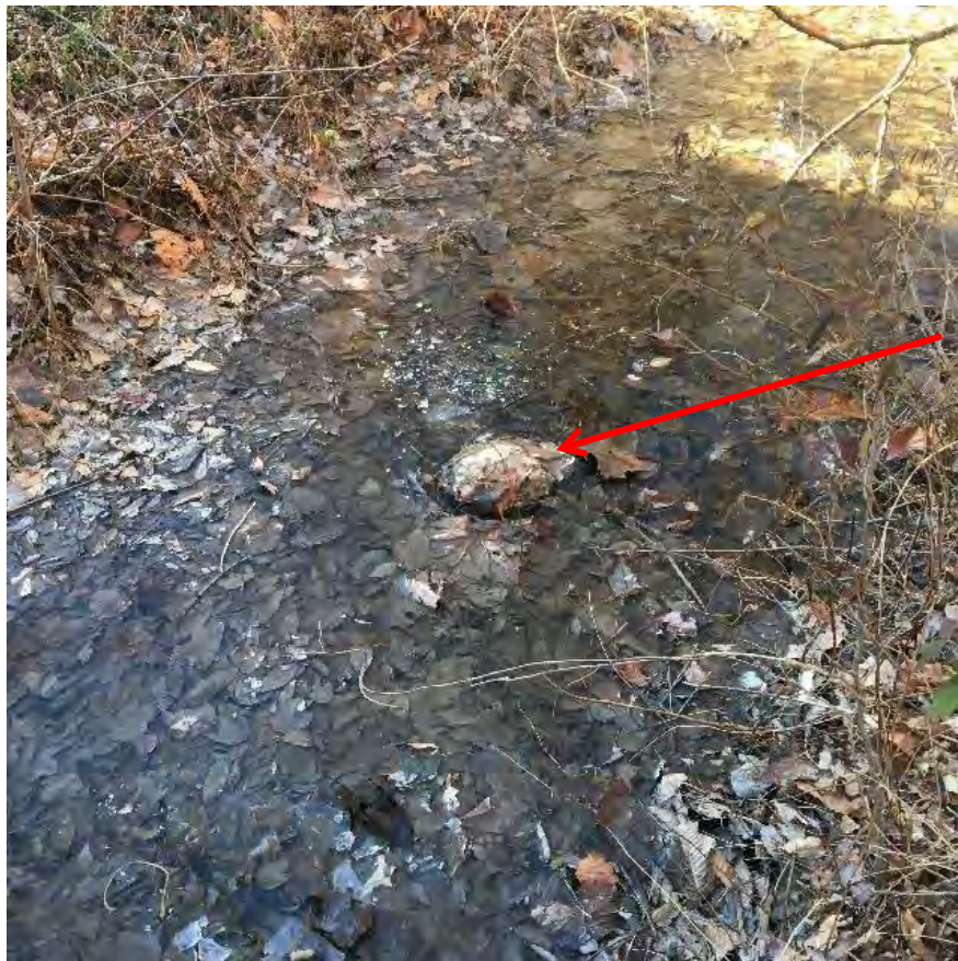
Ponding on BMP surface and observation well
