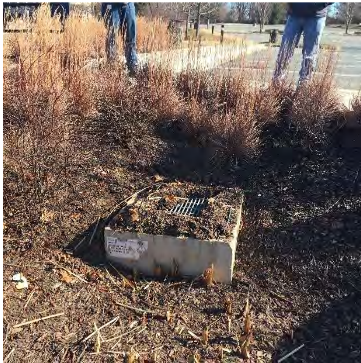
Overflow Device, Mulch on Inlet
