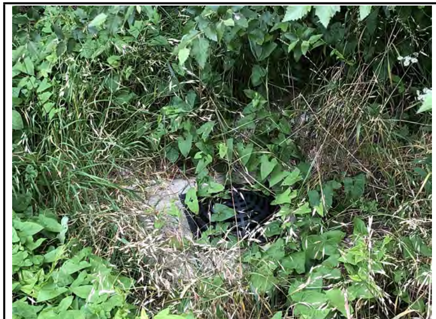
Photo #2: The outlet structure.
