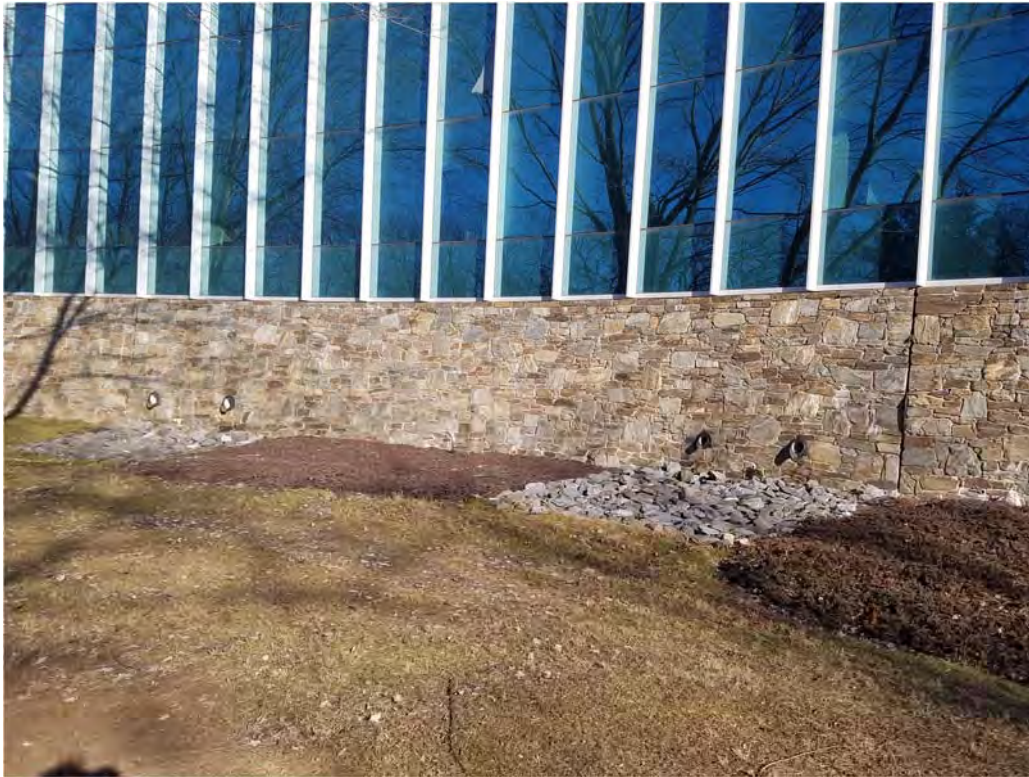
Inflow from roofdrain
