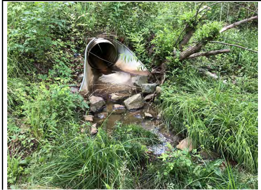
Photo #5: The second inflow culvert.
