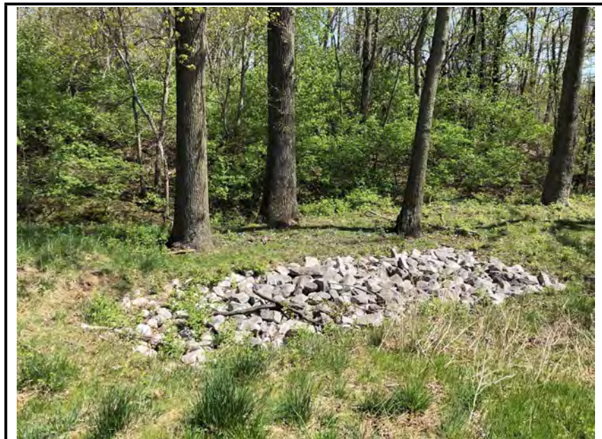
Photo #4: The riprap overflow channel.
