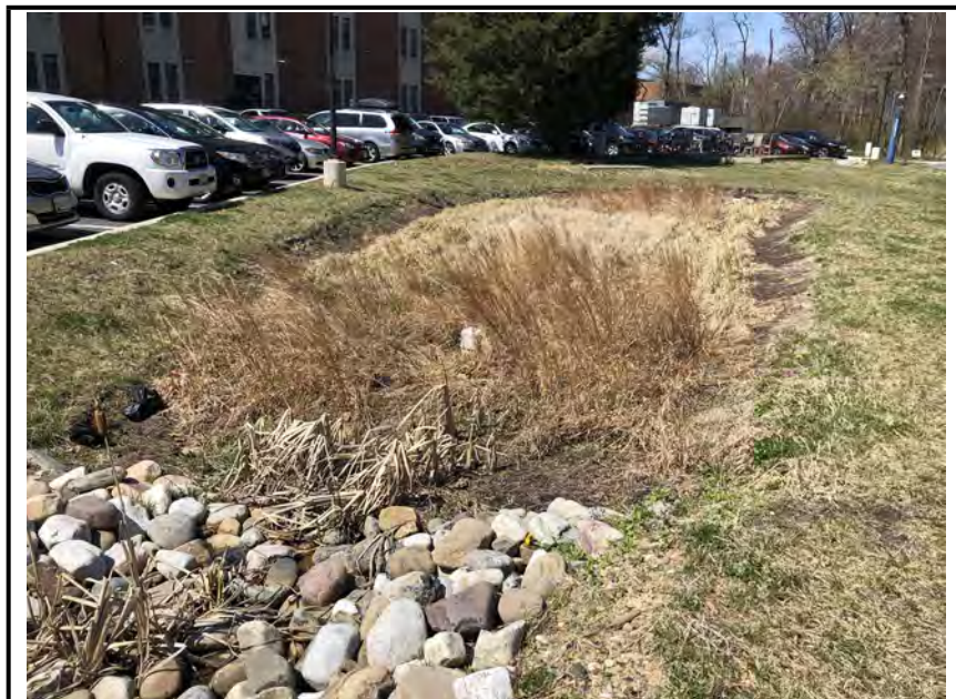
Photo #1: Inflow channel that leads to the facility.
