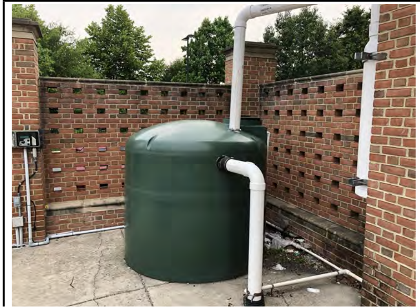
Photo #1: The rainwater harvesting facility.
