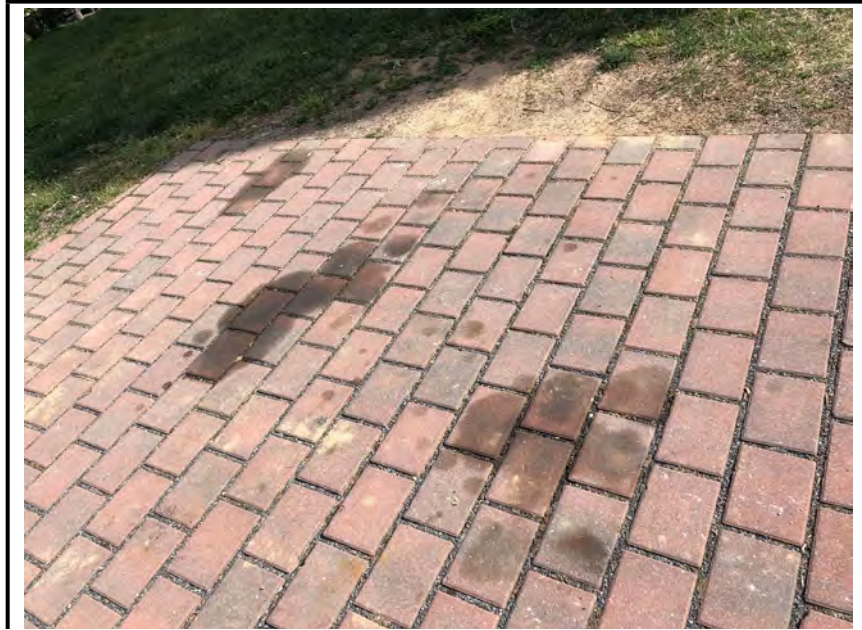
Photo #1: Oil spots on the pavers.
