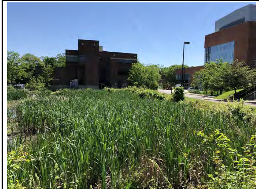
Photo #1: View into the facility from the outfall.
