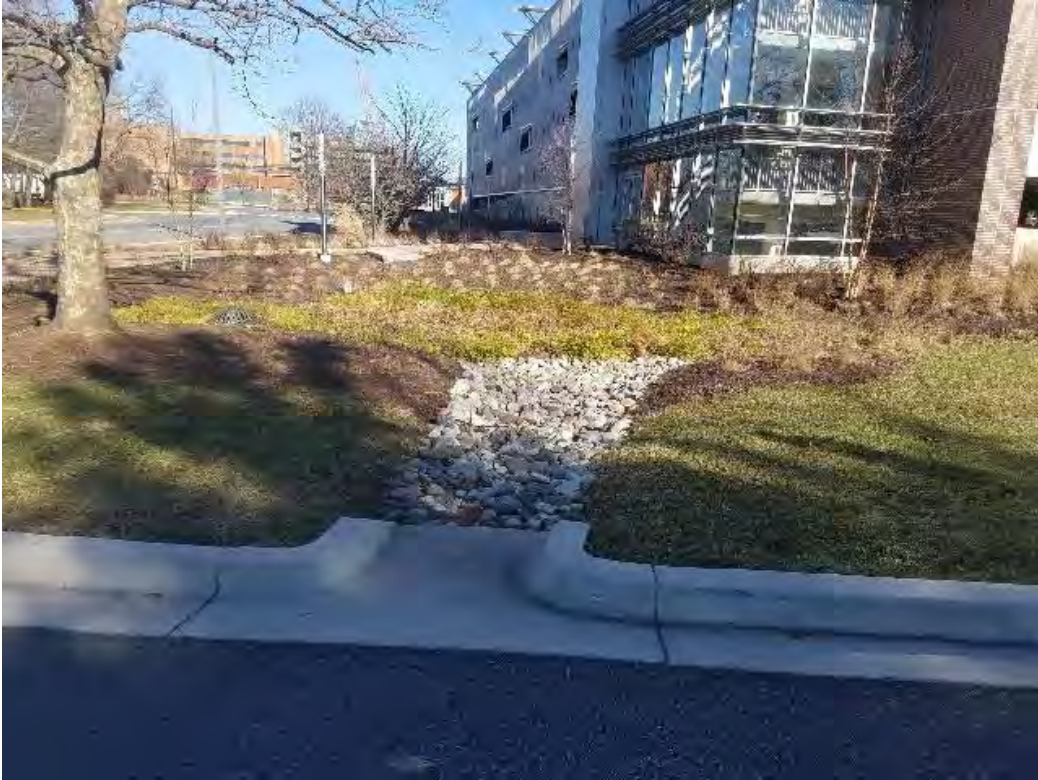
Inflow - Curb Cut
