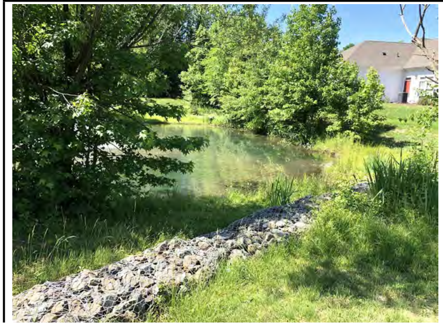
Photo #1: The gabion weir that separates the forebay from the facility.
