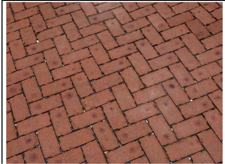
Photo #1: Semi-clogged pores in pavement.
