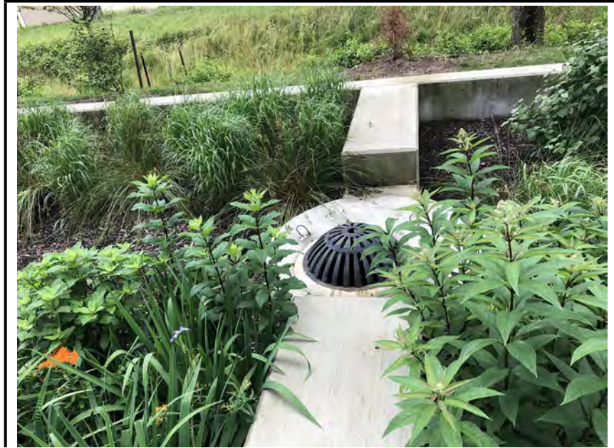
Photo #1: The riser outlet structure shared with CH-1
