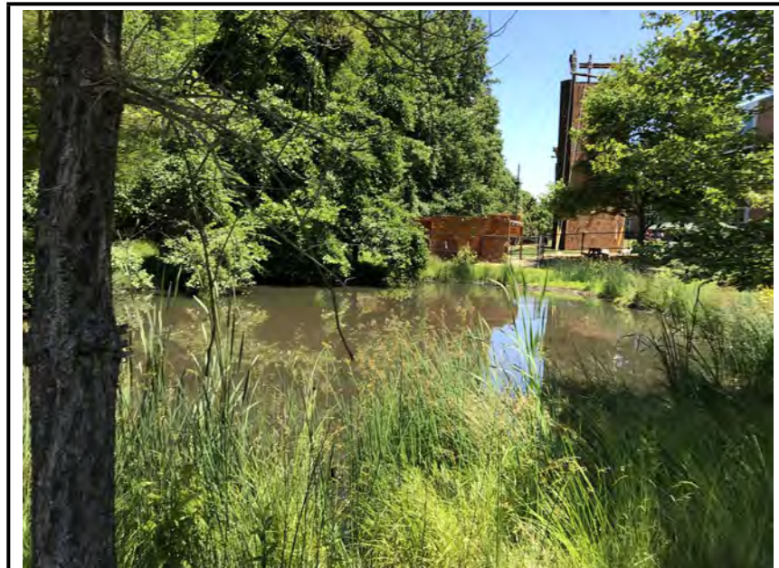
Photo #2: View into the facility.
