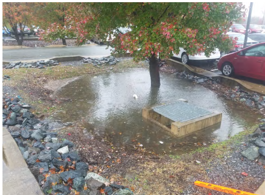
Figure 3 - Bioretention facility during rain event
