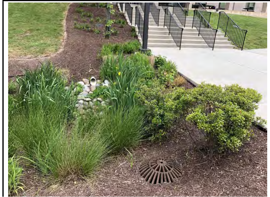
Photo #1: Outlet structure flush with the mulch elevation.
