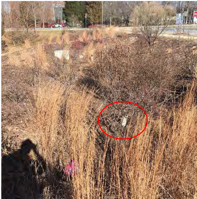
Overall - Facing North, Cleanout
