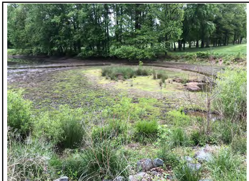
Photo #4: Filter area of the facility.
