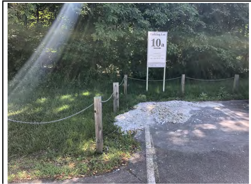
Photo #1: Gravel that is blocking the non-structural practice.
