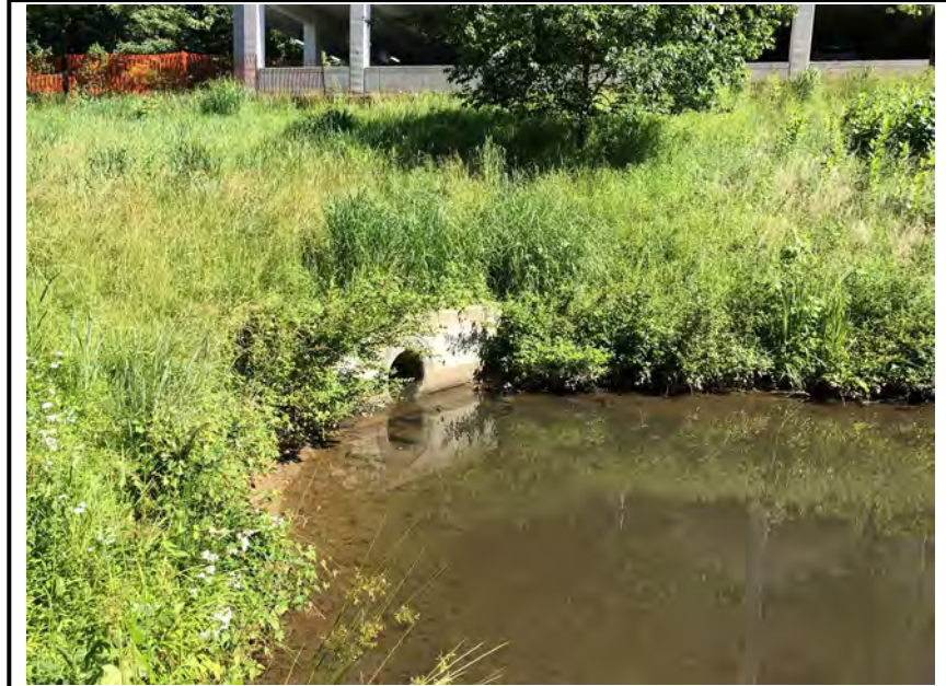
Photo #3: The concrete inflow culvert.
