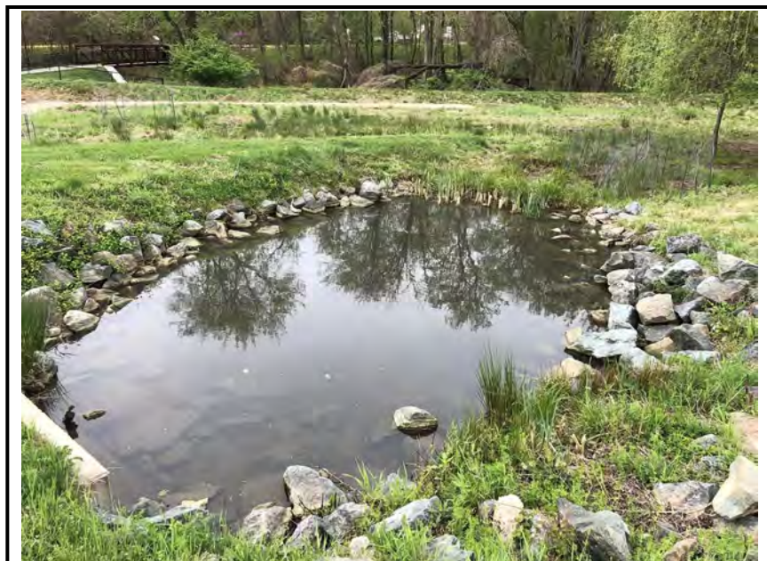
Photo #6: Stagnant water in the forebay.
