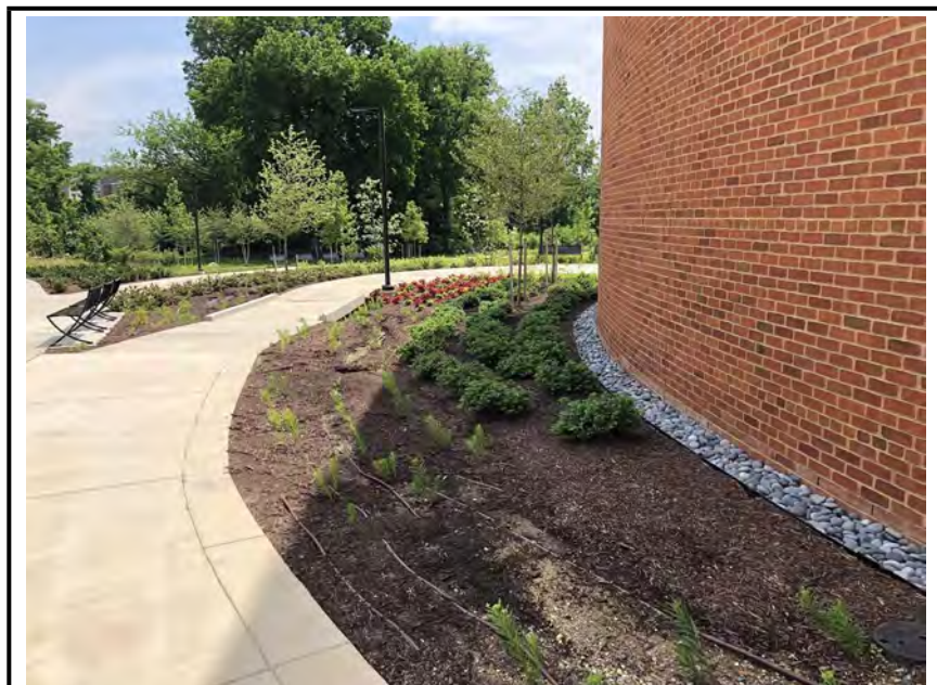
Photo #2: Exposed irrigation lines in the inflow swale.
