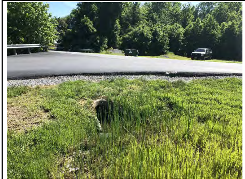
Photo #1: The inflow culvert to the facility.
