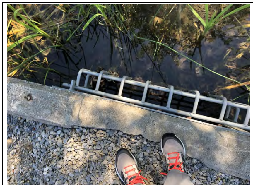
Photo #4: The outlet structure.
