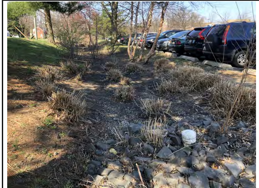
Photo #3: View onto the filter area.
