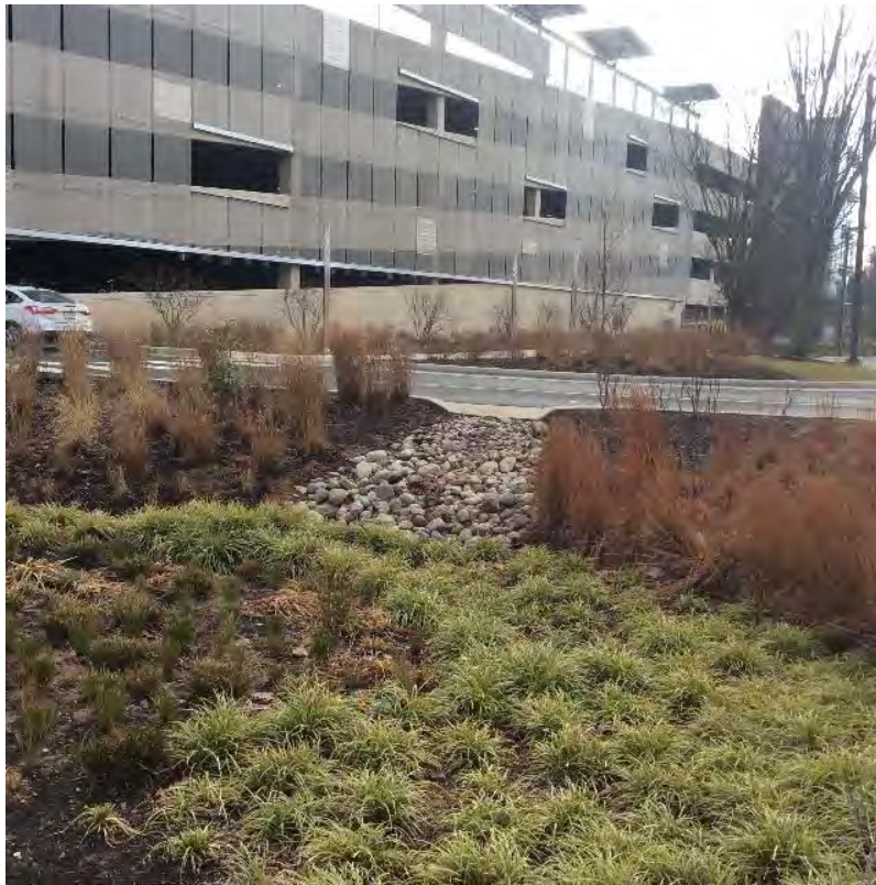
Inflow - Curb Cut and unknown pipe
