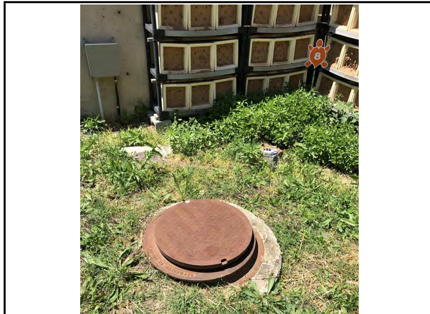
Photo #3: The manhole that leads to the cistern.
