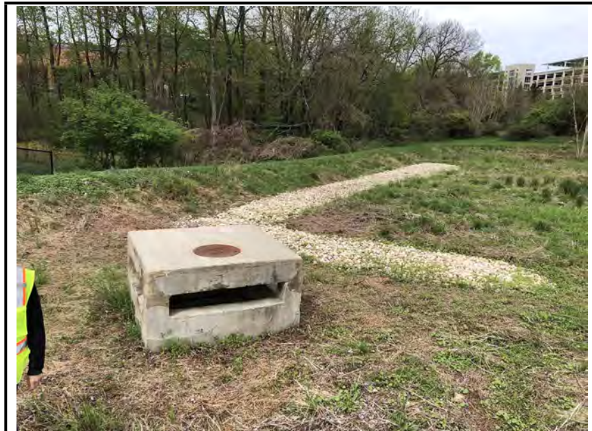
Photo #2: Outlet structure.
