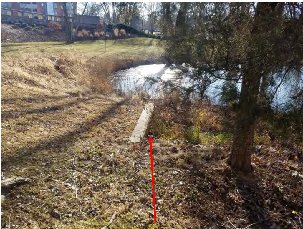
Inflow from pipe, partially buried
