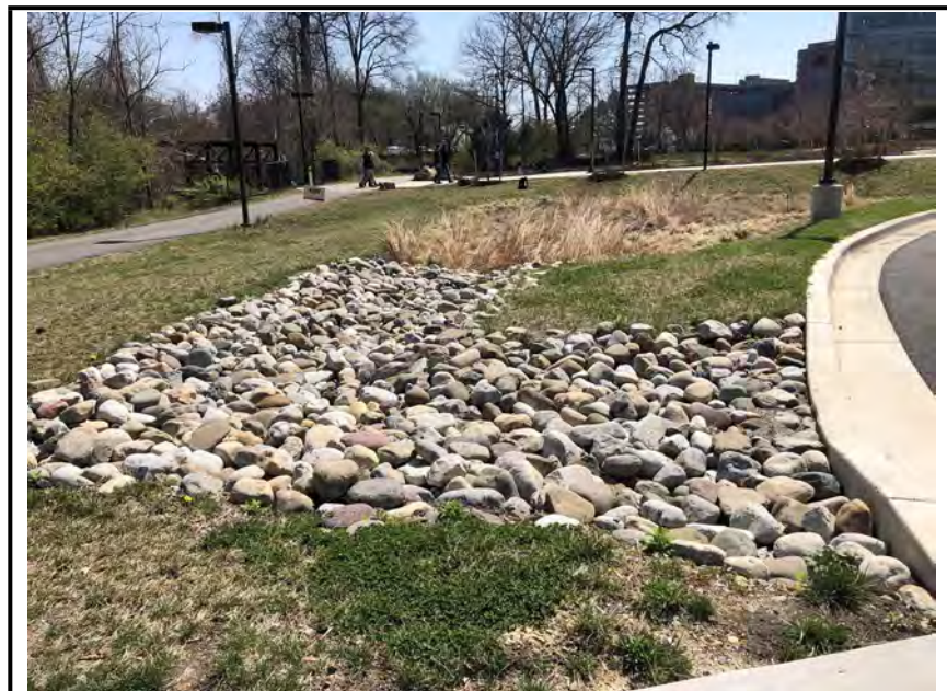
Photo #4: The riprap channel that serves as pretreatment.
