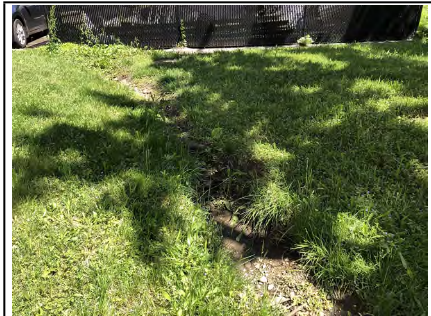
Photo #2: Erosional gully that leads into the facility inlet.
