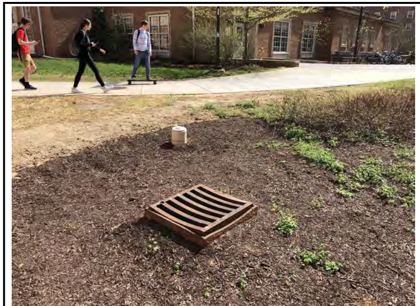
Photo #2: The riser outlet structure.
