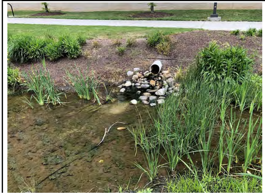
Photo #1: An eroded and algae-covered inflow pipe.
