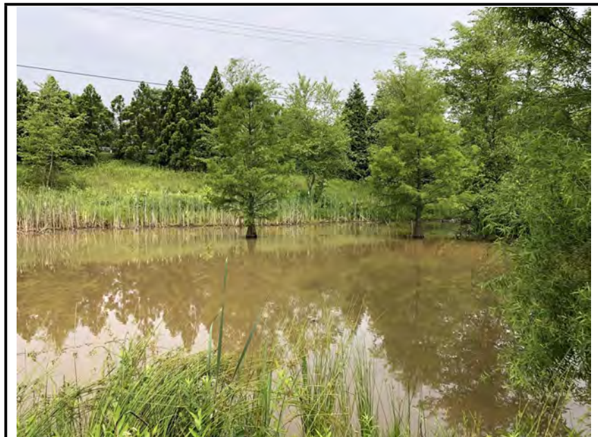
Photo #4: Trees and low flow in the forebay.
