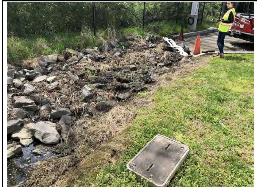
Photo #3: The riprap inflow channel.
