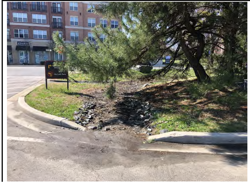
Photo #1: One of the curb cuts that leads to the facility.
