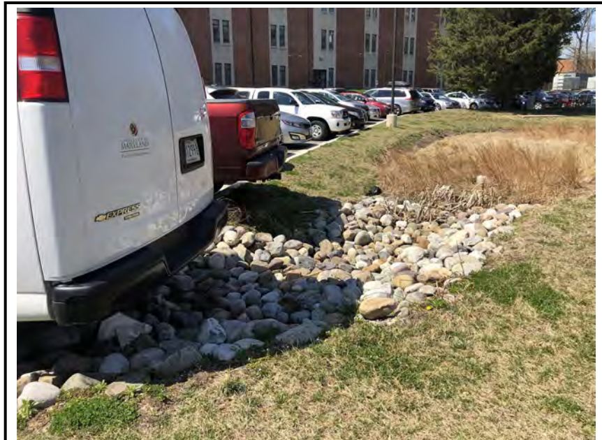
Photo #1: Inflow channel that leads to the facility.
