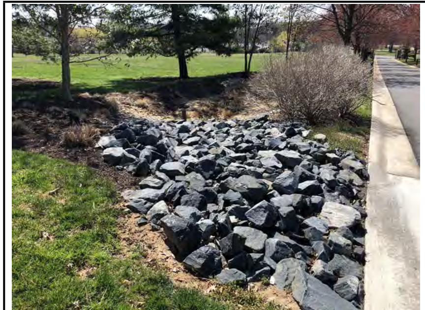
Photo #3: The riprap lined curb cut.
