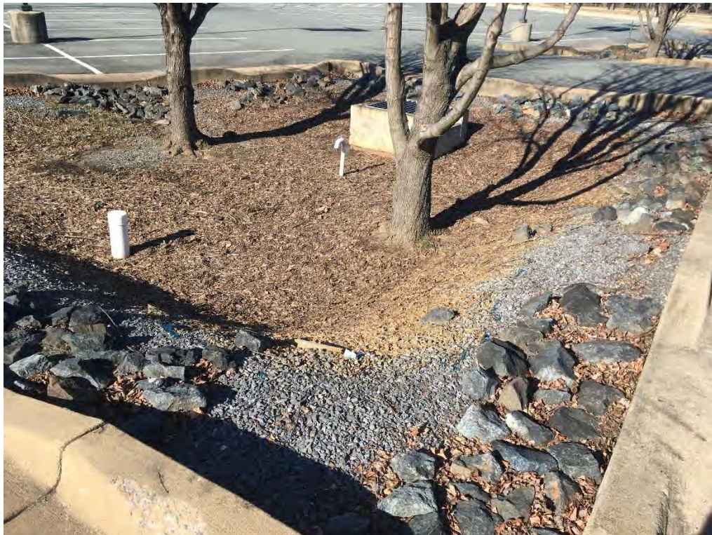
Overall, Facing North
