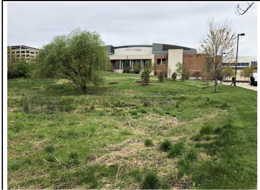
Photo #1: View into facility.
