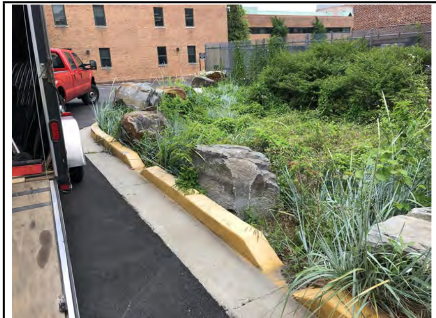
Photo #2: Curb cuts that lead into the facility.
