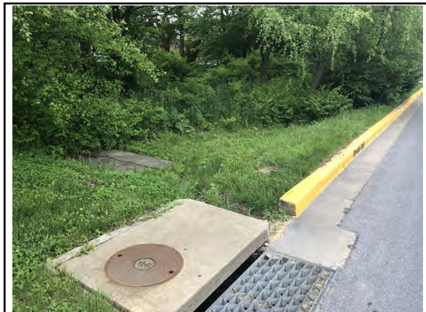
Photo #2: Inlet next to the inflow curb cut.
