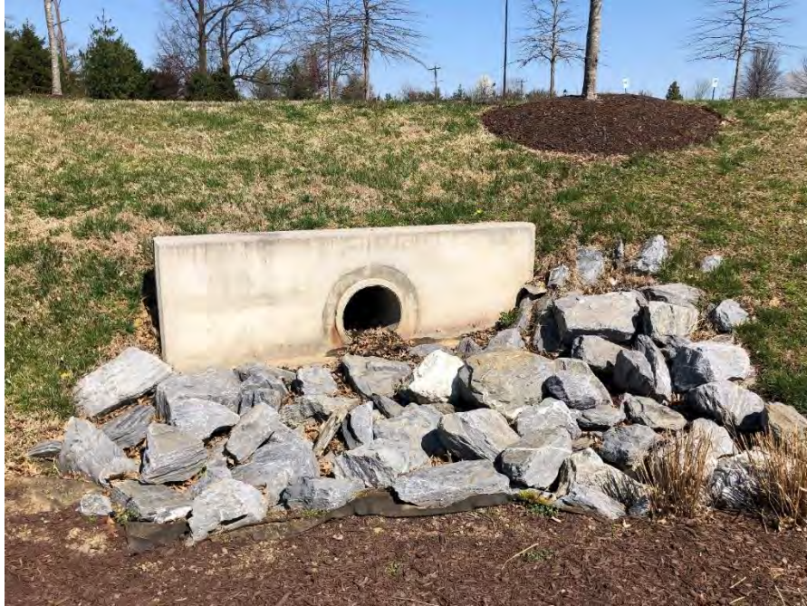
Photo #3: Inflow culvert into the facility.
