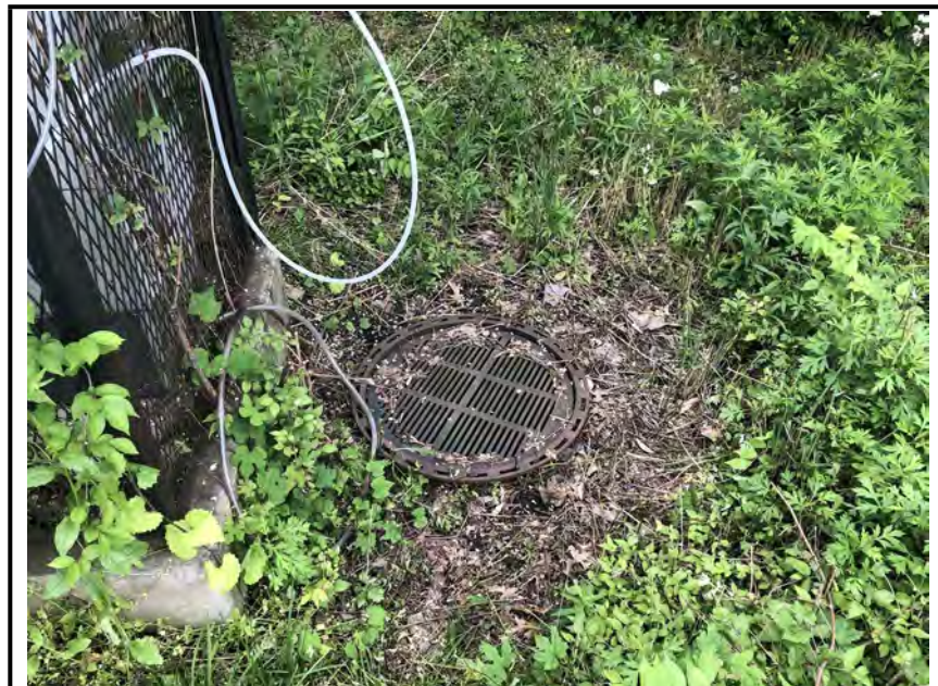
Photo #2: Outlet structure next to the inflow channel.
