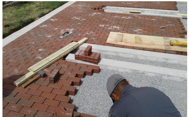
Staff Building a Pervious Paver Bike Parking Pad
