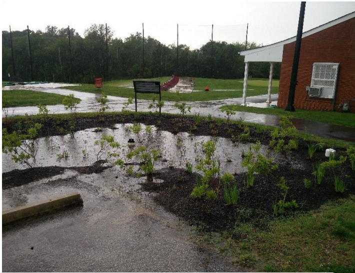
Stormwater from a parking lot ponding in a newly built bioretention facility
